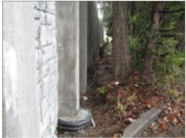
Close placement of noise wall adjacent to mature trees.
