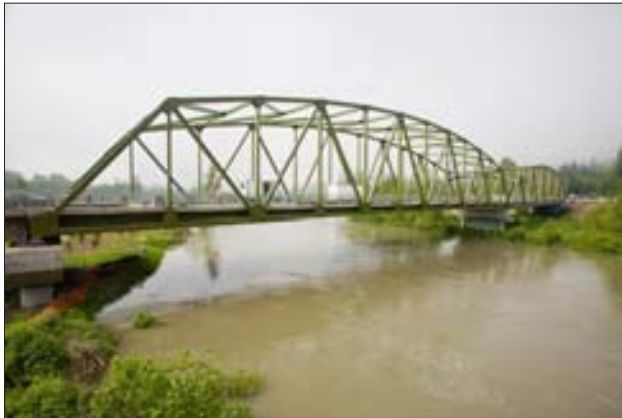
Tolt River Bridge – King County
