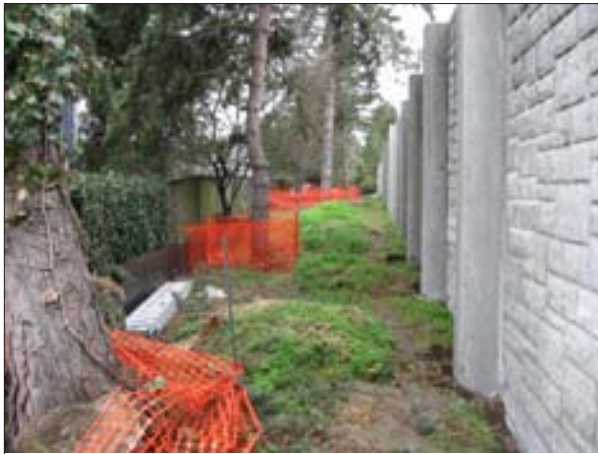
Mature trees protected during noise wall construction.
