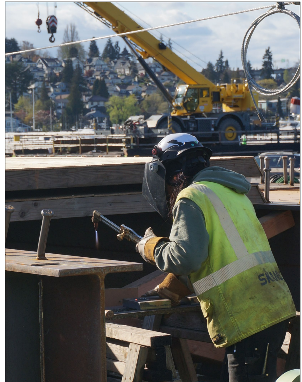
A welder joins beams to make a new SR 520 off-ramp (April 2026)
