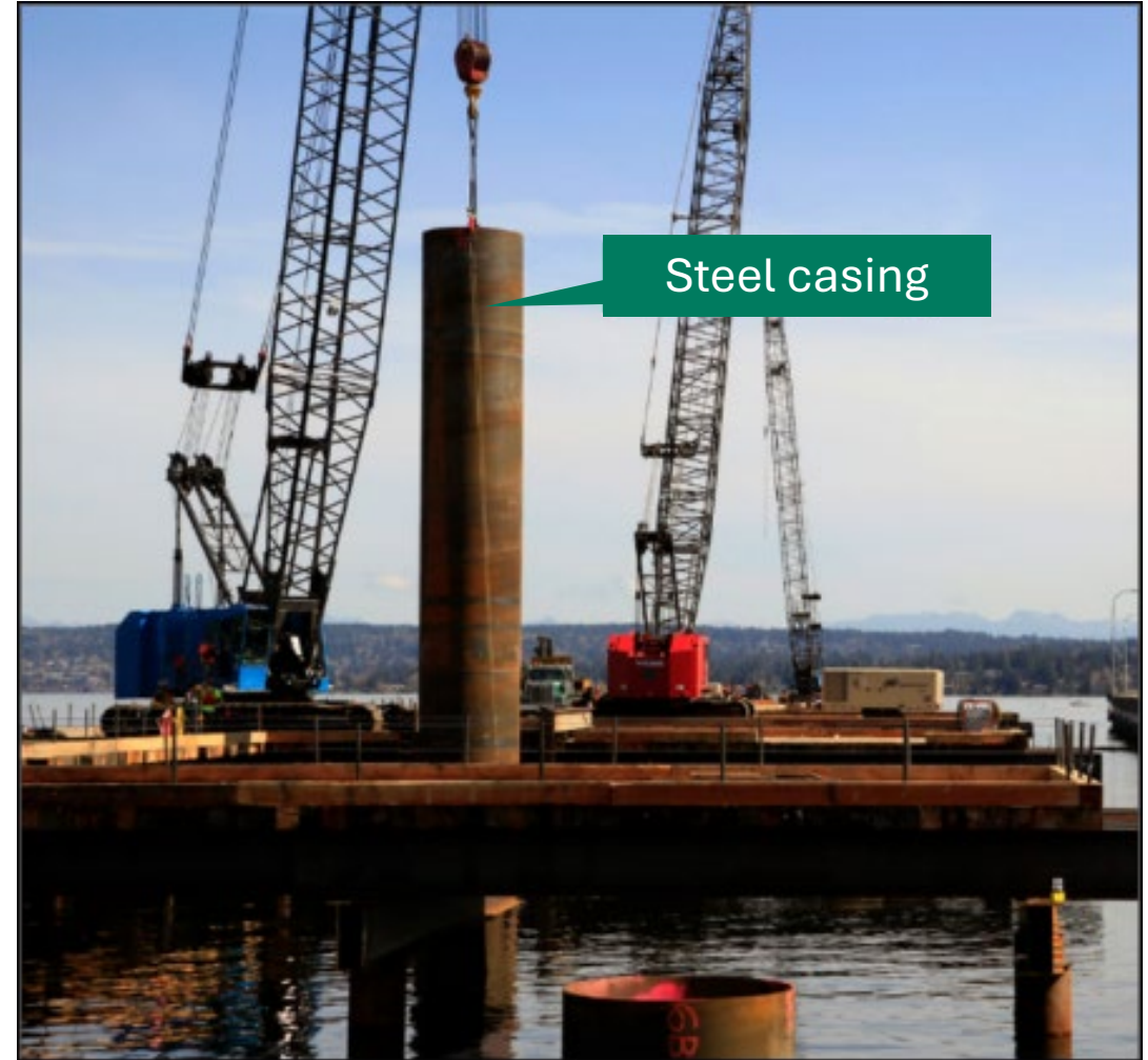
An example of crane lowering a casing section into place.
