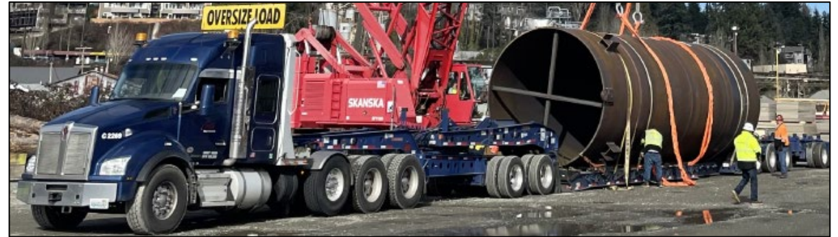
A crane loading a section of casing onto a truck.
