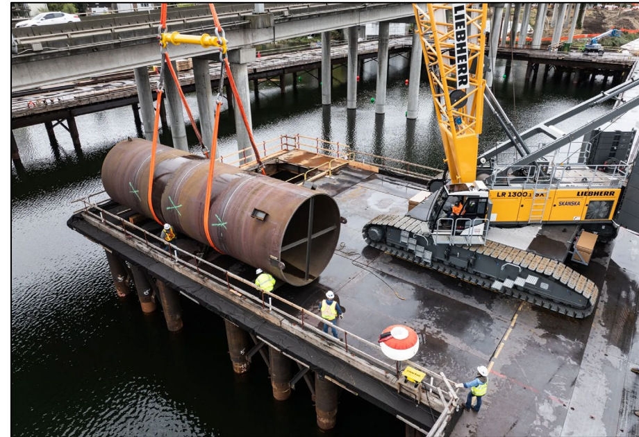
A crane places a section of casing on the trestle (April 2026)
