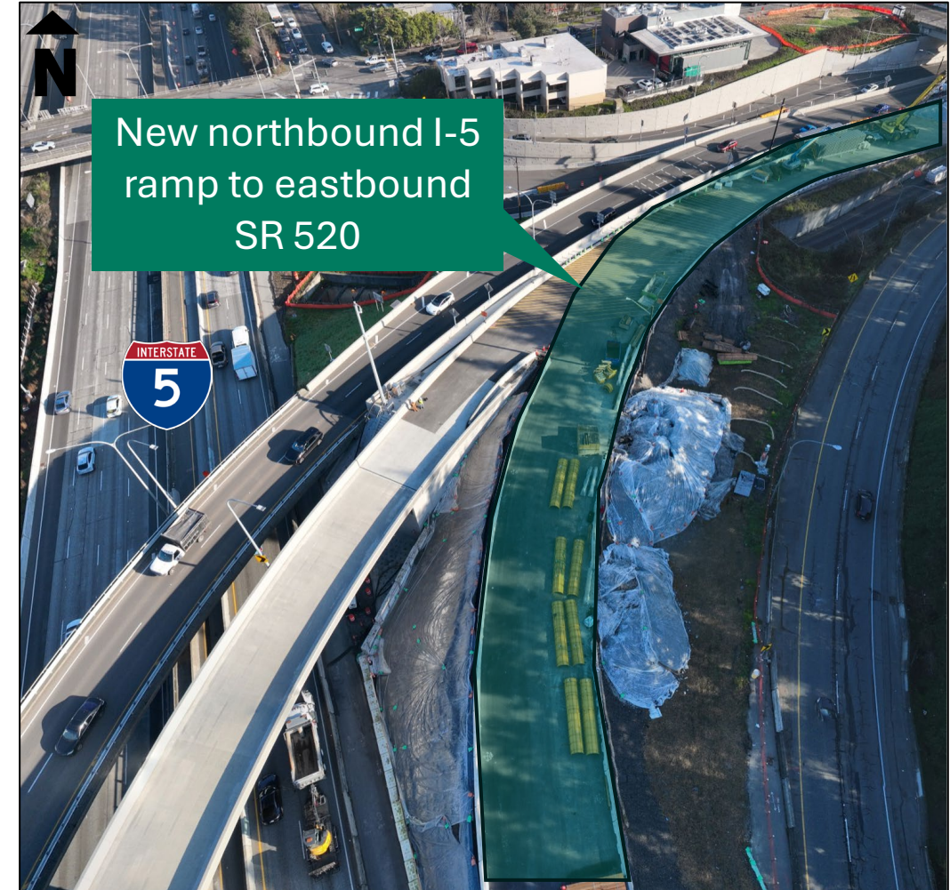
Aerial view of the I-5/SR 520 interchange and the new northbound I-5 ramp to eastbound SR 520.
