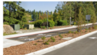
Separated Two-Way Bike Lane on one side of the street, with sidewalks on both sides of the street, all separated from vehicle traffic.
