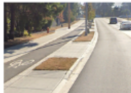
Bike Lanes and Sidewalks running alongside one another in the direction of vehicle travel, separated from vehicles.
