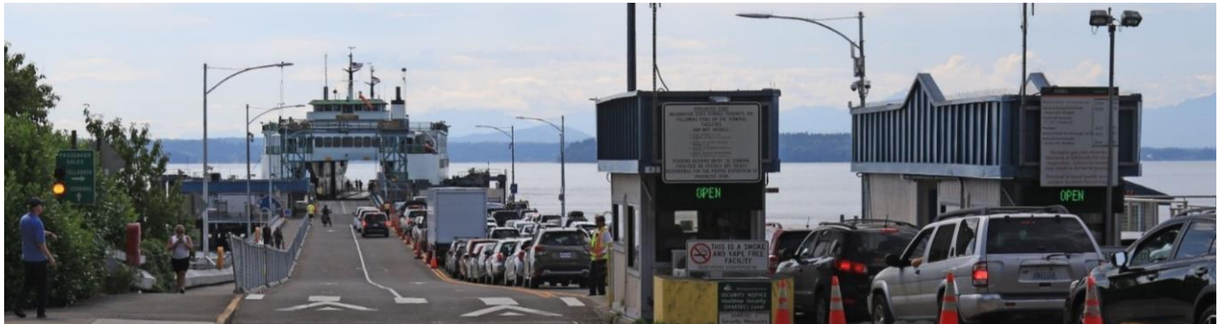
Figure 3. Existing Fauntleroy Ferry Terminal Ticketing and Loading Operations
