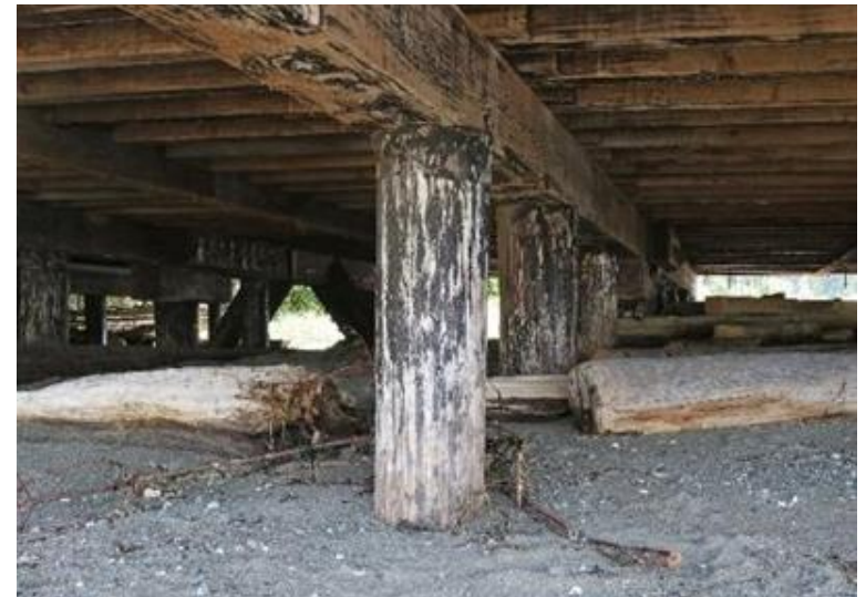
Figure 6. Creosote-treated Timber Piles Supporting the Existing Fauntleroy Ferry Terminal Trestle
