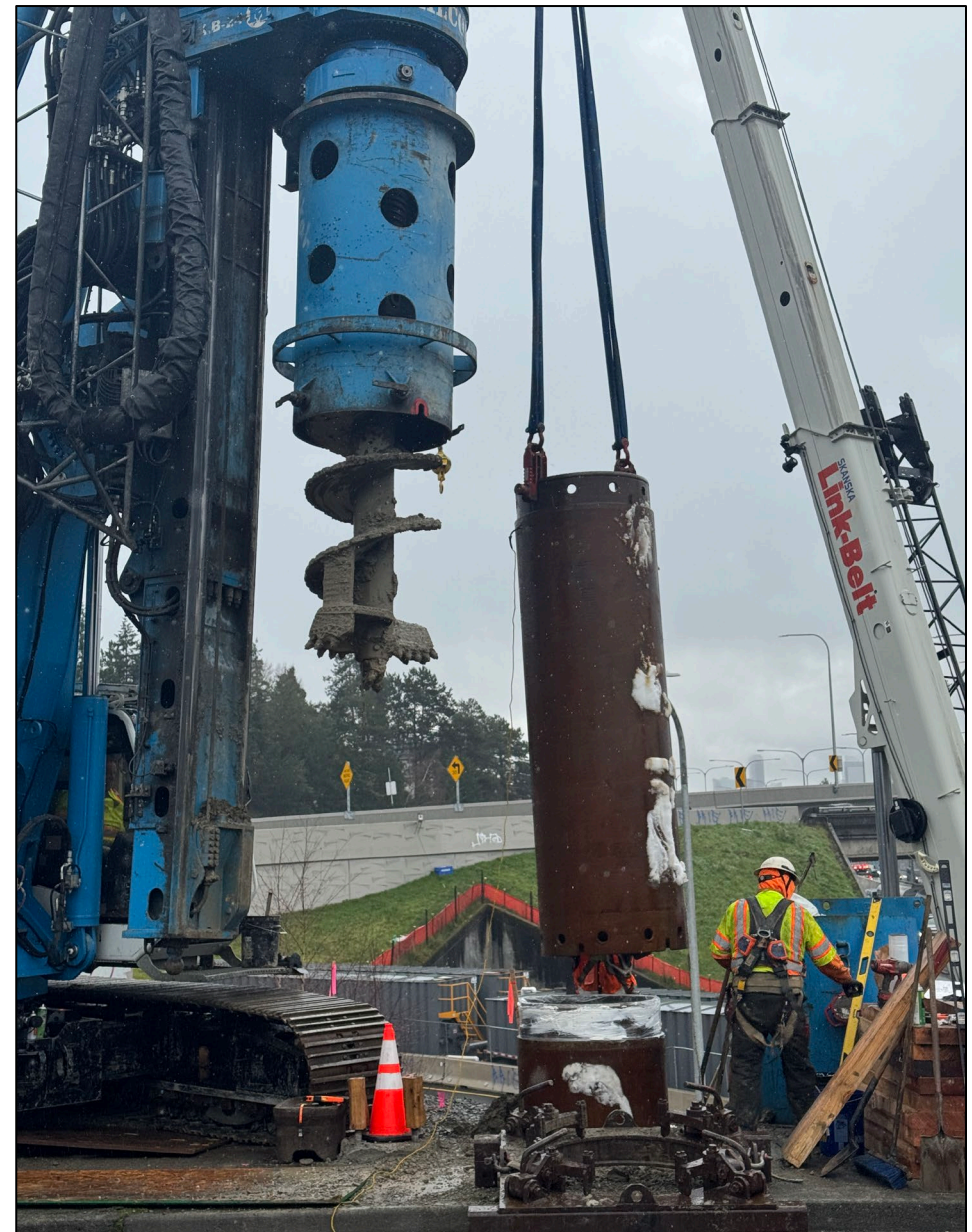
Crews installing piling along East Roanoke Street
