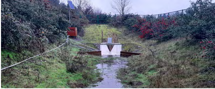
Figure 3 Vancouver effluent flume and monitoring station
