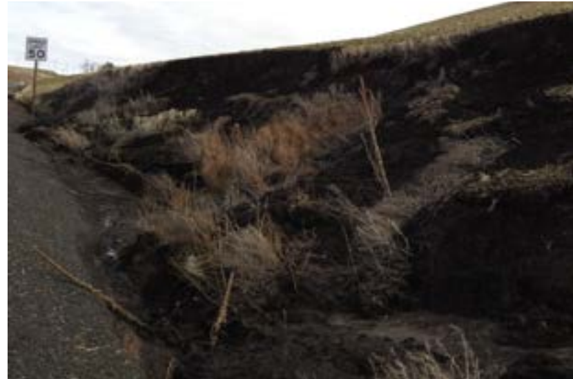
Figure 2. Farming too close to the edge of the roadway can cause erosion as seen at this site identified on SR 272 during a highway evaluation required by a TMDL.
