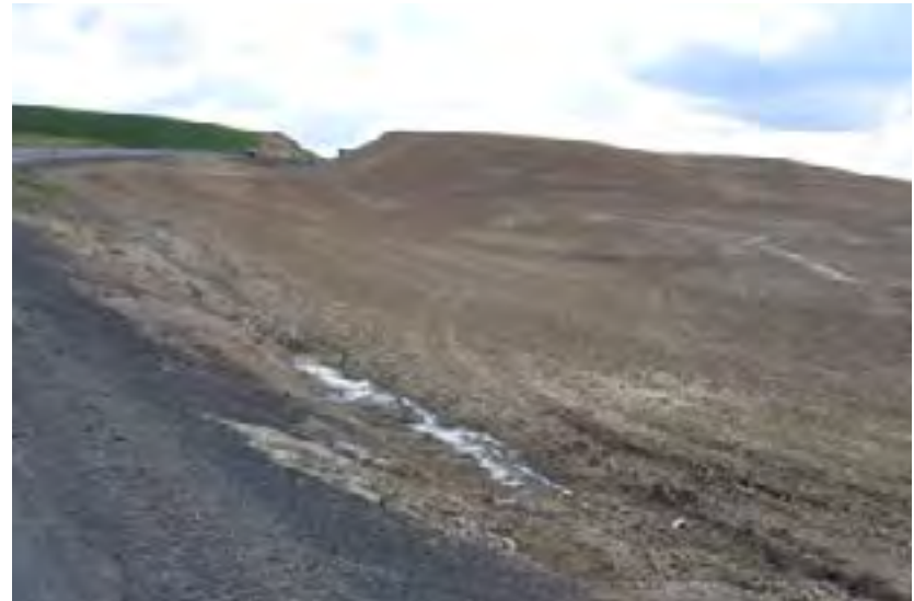
Figure 2. WSDOT works with Ecology to identify priority locations for remedying erosion problems associated with farming activity in some eastern Washington watersheds. Chronic erosion from farming activity is an ongoing maintenance and water quality challenge, as seen at this location on SR 27 within the Hangman TMDL.
