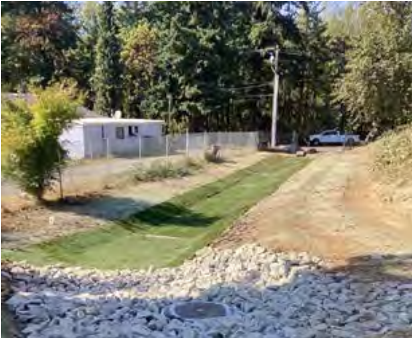
Figure 5. A bioswale near Salmon Creek is reconstructed by Southwest Region Area 1 crews.
