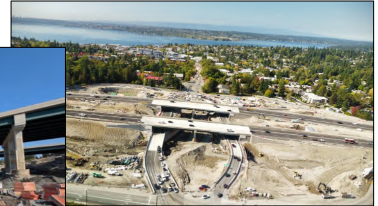
Aerial view looking west
