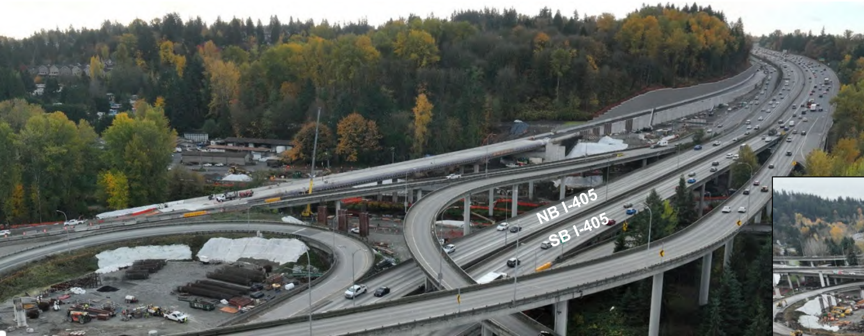
Aerial view of I-405/SR 522 interchange looking southeast
