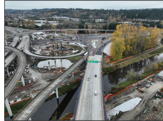
New bridge deck over Sammamish River near Woodinville Drive
