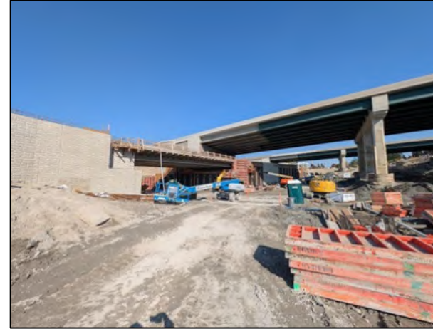
Excavation under new bridge decks
