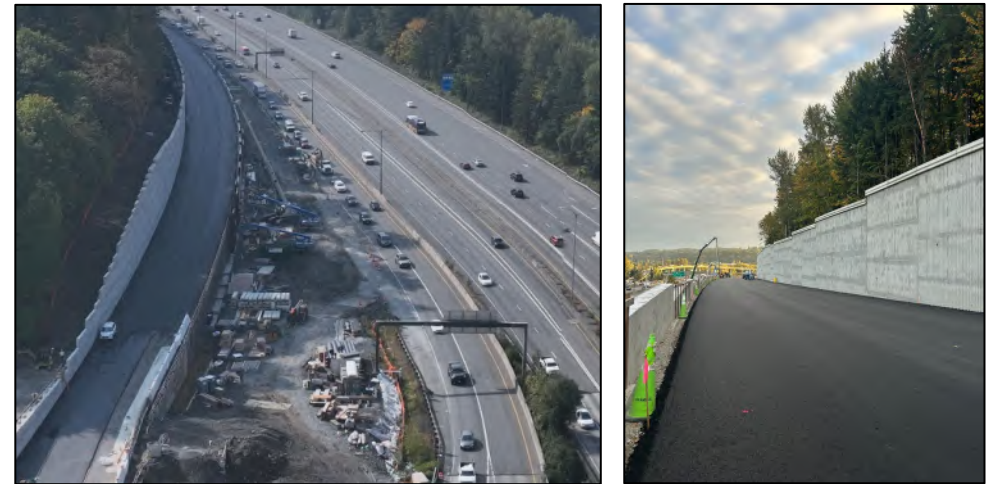
Retaining walls anchored to the surrounding soil using steel rods
