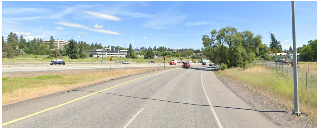
US 2 to I-90 ramp before installation
