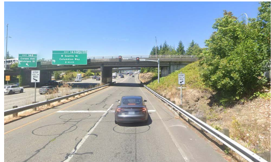
Northbound Swift Ave after installation of ramp meter
