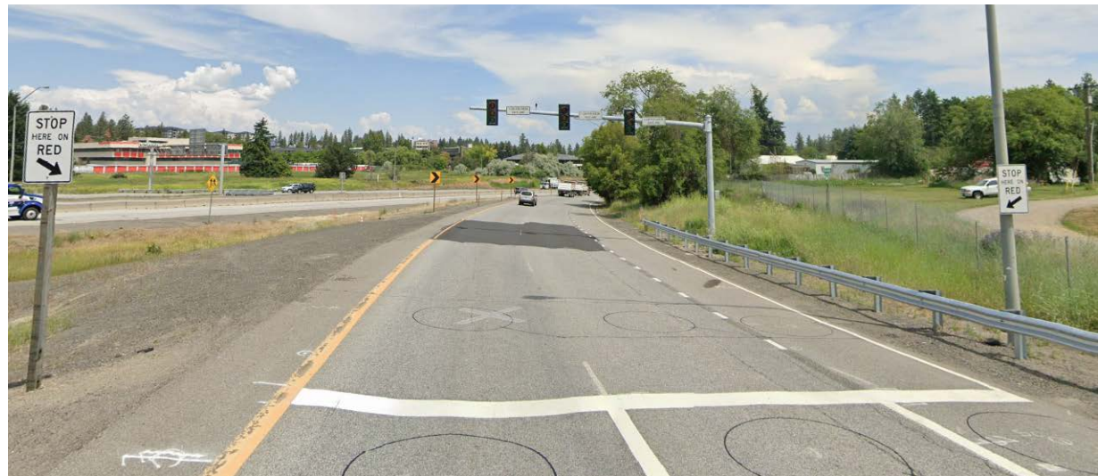
US 2 to I-90 ramp after installation of ramp meter
