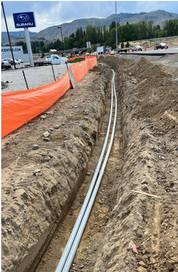
Installation of conduit on the side of SR 285 while under construction
