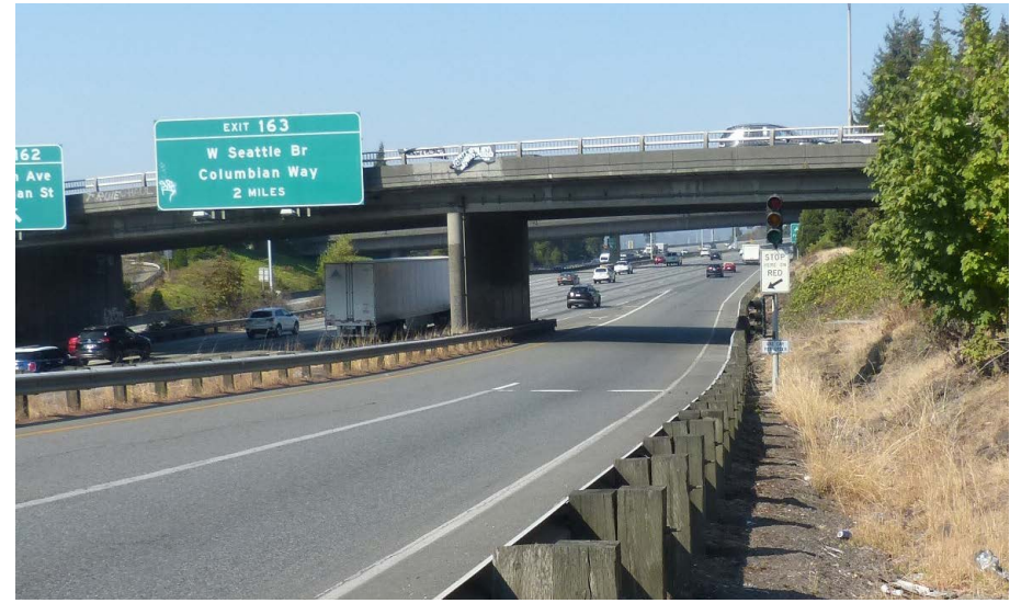
Northbound Swift Ave before installation of ramp meter
