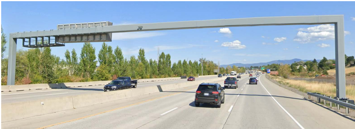
Eastbound I-90 before VMS installation
