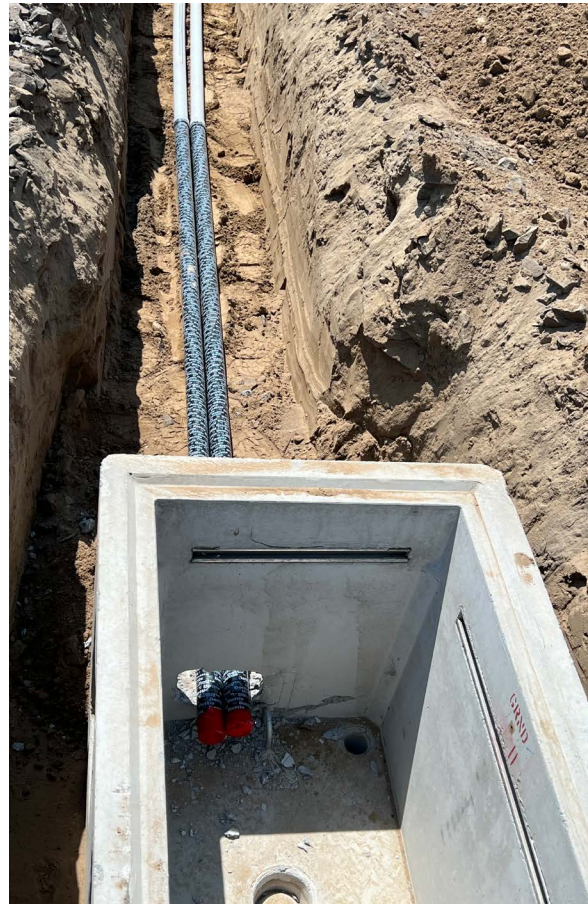
Installing conduit at SR 285 before the excavation is filled
