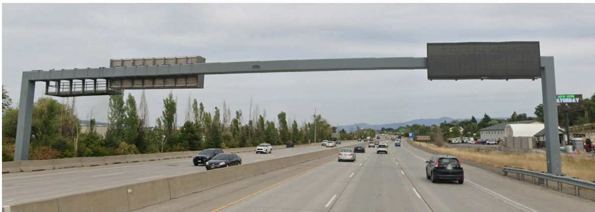
Eastbound I-90 after installation
