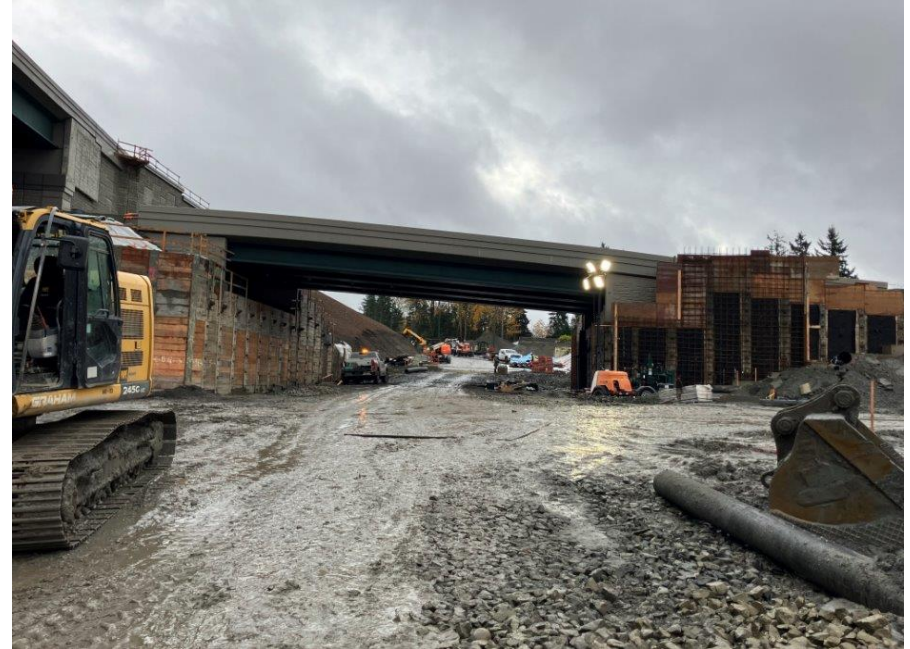
In progress excavation under the I-405 lanes
