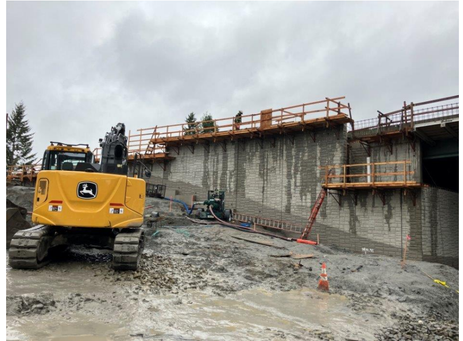
The excavation in progress under the I-405 bridges.
