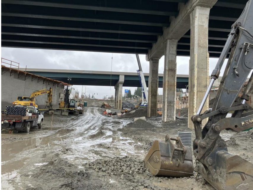
Northeast 85th Street excavation under NE 85th Street.
