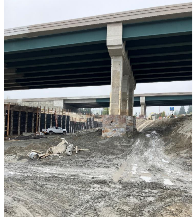
The excavation in progress under the I-405 bridges.
