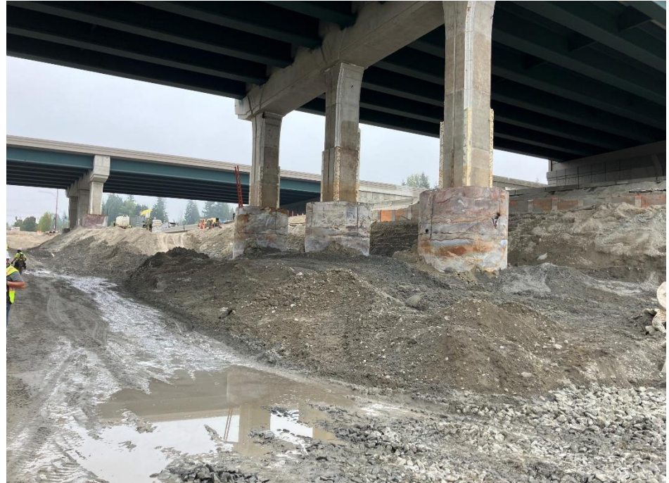
In progress excavation under the I-405 lanes
