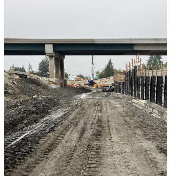
In progress excavation under the I-405 lanes
