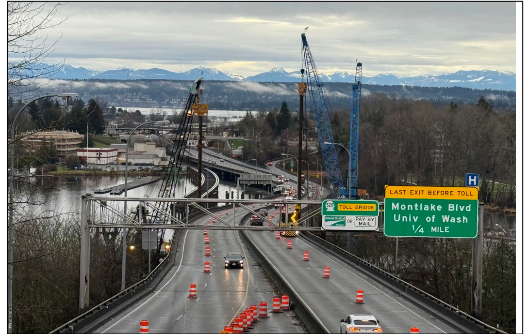
Recent weekend single-lane closures on SR 520.
