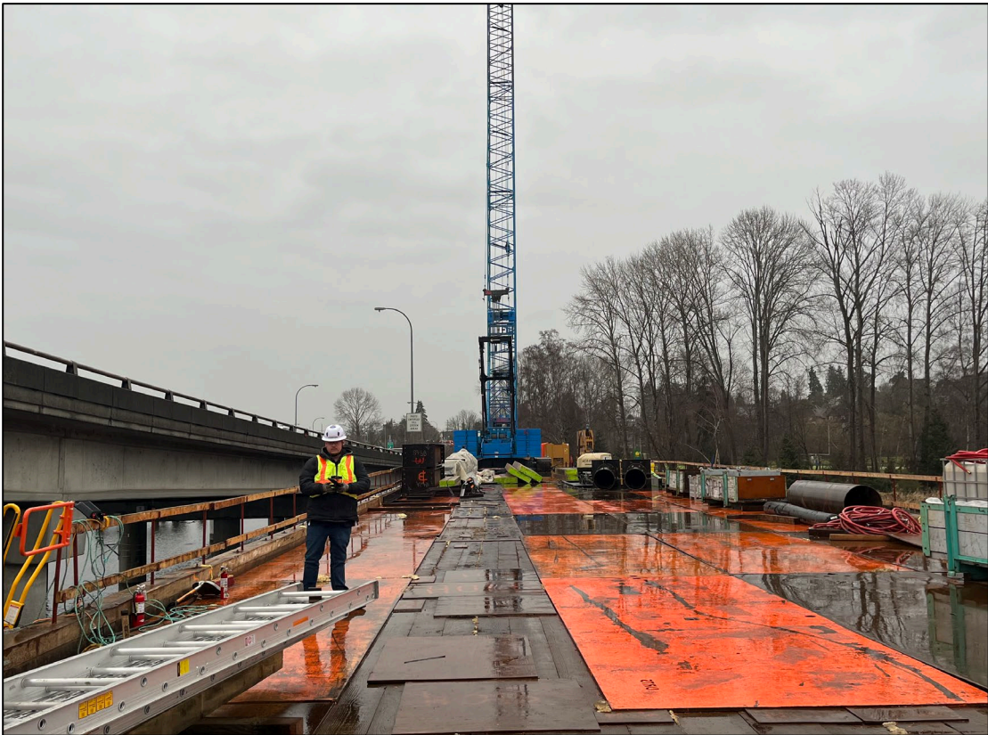
Crews installing decking on the temporary work trestle.
