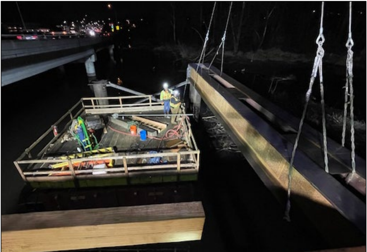
Crews installing decking on the temporary work trestle.
