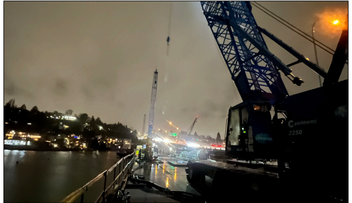
Crews constructing the work trestle platform at night.
