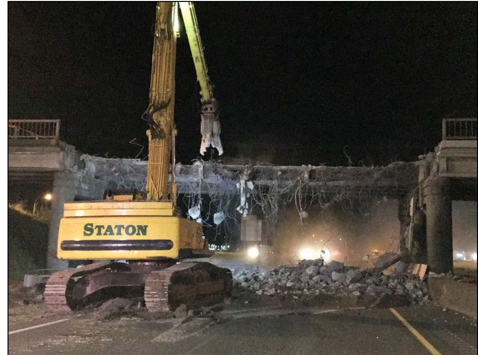
Removing concrete structures over SR 520.
