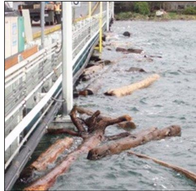
Existing dock during a high tide
