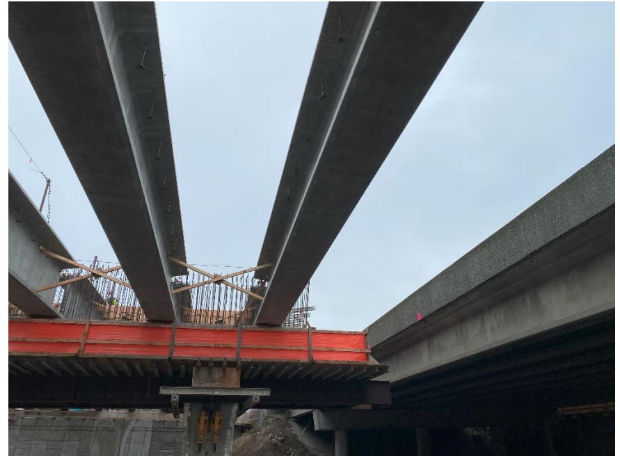
Girders for new northbound I-405 bridge.
