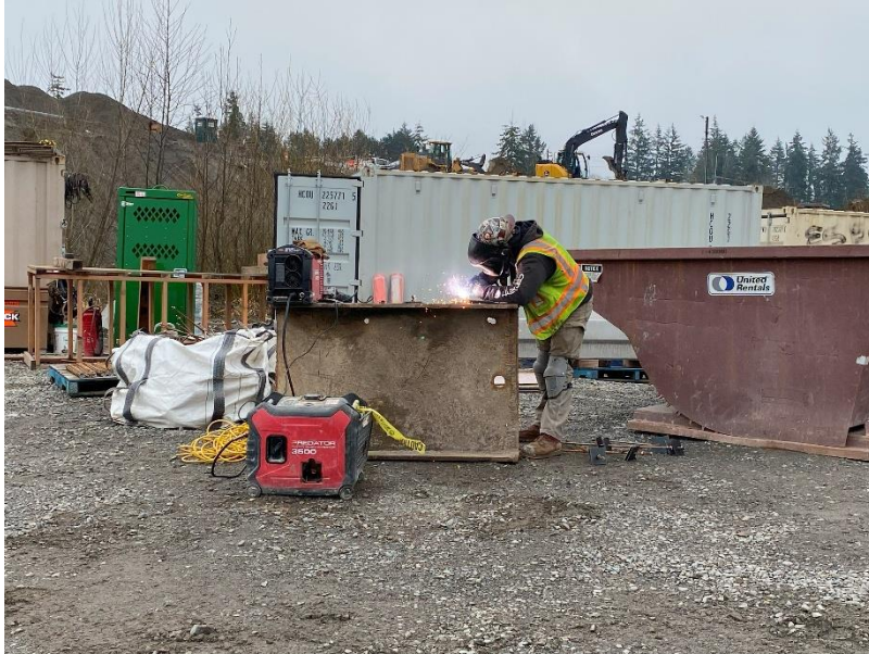
Crews preparing for the girders on the I-405 bridge.
