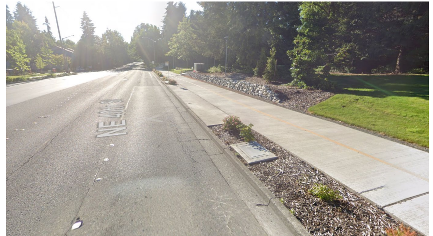
Local routes (KC Metro) on NE 40 th St (Redmond, WA)
