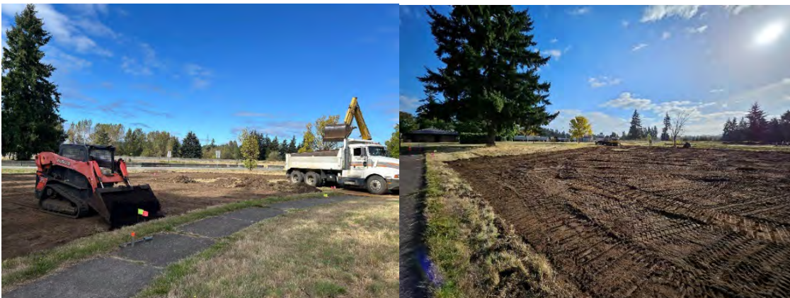
Figure 5-6: Cleared and grubbed land.
