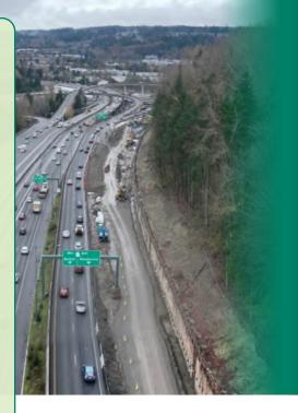
Looking northbound on I-405 toward the SR 522 interchange, crews built a massive retaining wall to make space for the dual ETL system. Crews built 43,500 square feet of permanent wall and excavated 100,000 cubic yards of dirt this year on the project.
