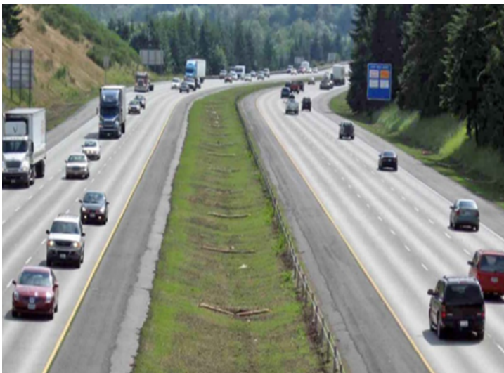
Compost amended vegetated filter strip
