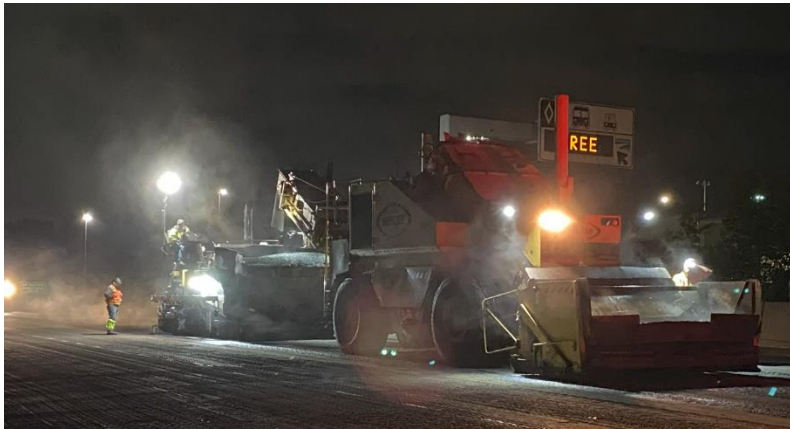
Nighttime paving work on southbound SR 167.
