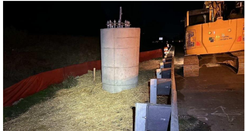
Concrete column foundation to support a new toll gantry.
