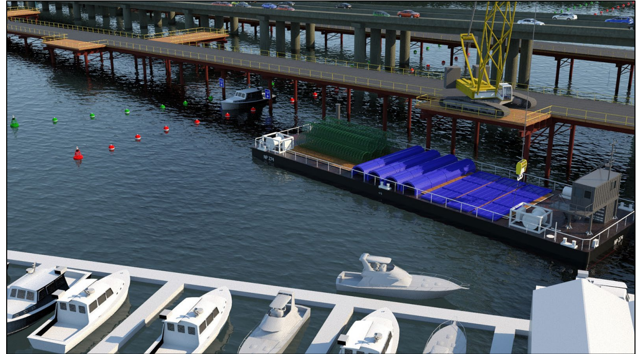
Rendering of the temporary work trestle in Portage Bay.
