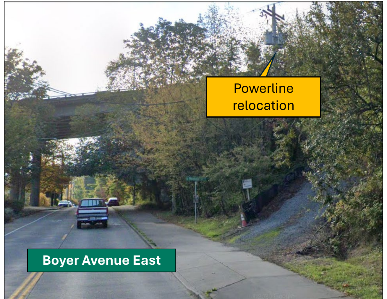
Location of the powerline near the WSDOT access road on Boyer Avenue East.
