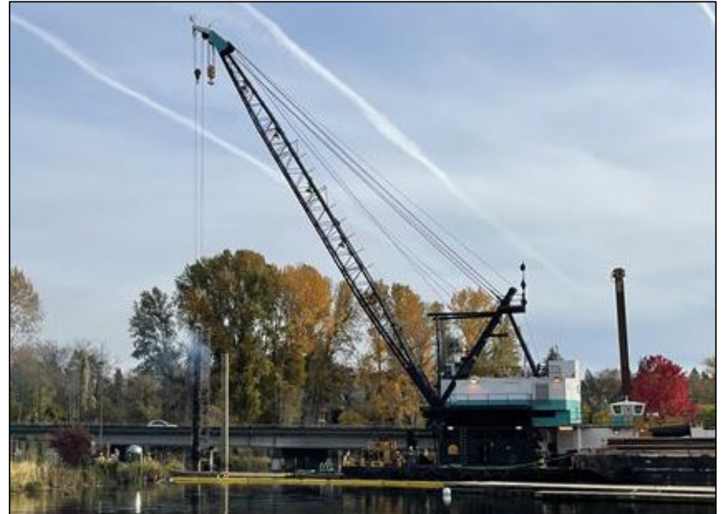
The barge used for piledriving in Portage Bay.
