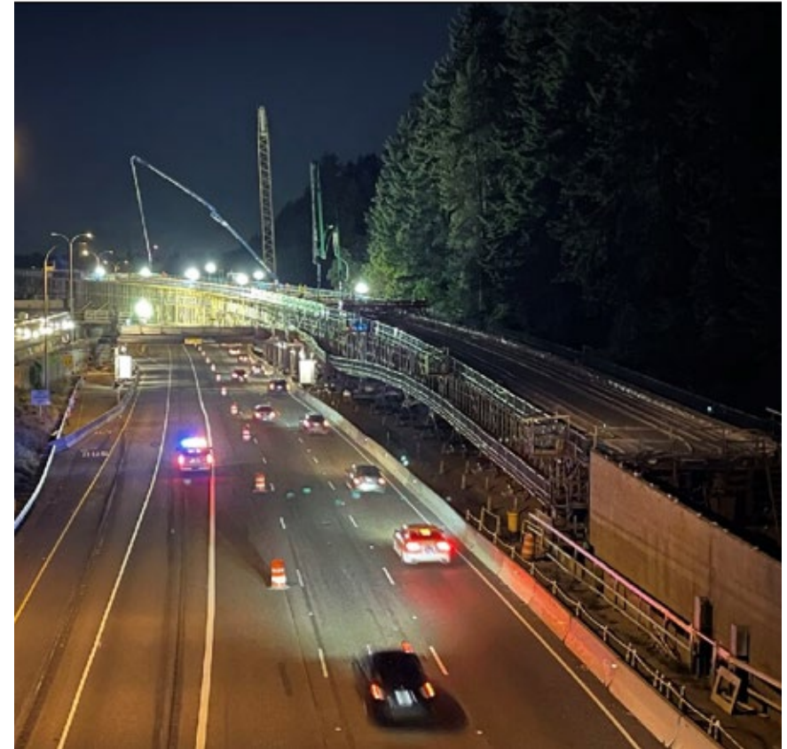
Crews may pour concrete during nighttime work.
