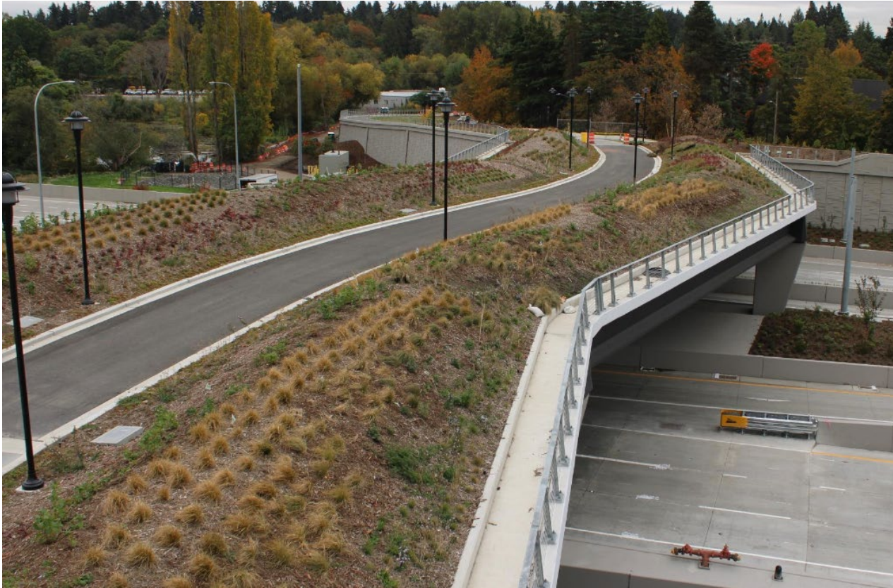
Bicycle and pedestrian bridge deck (October 15)
