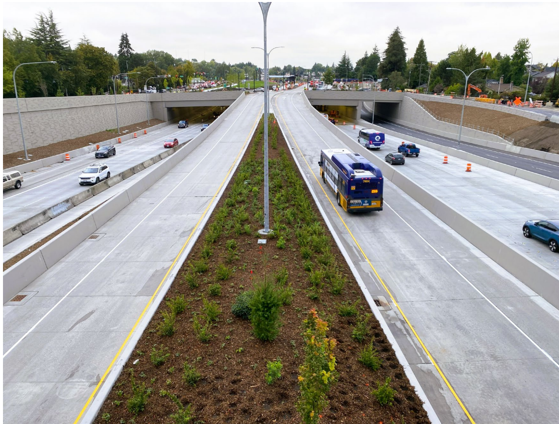
HOV direct access ramps (September 17)
