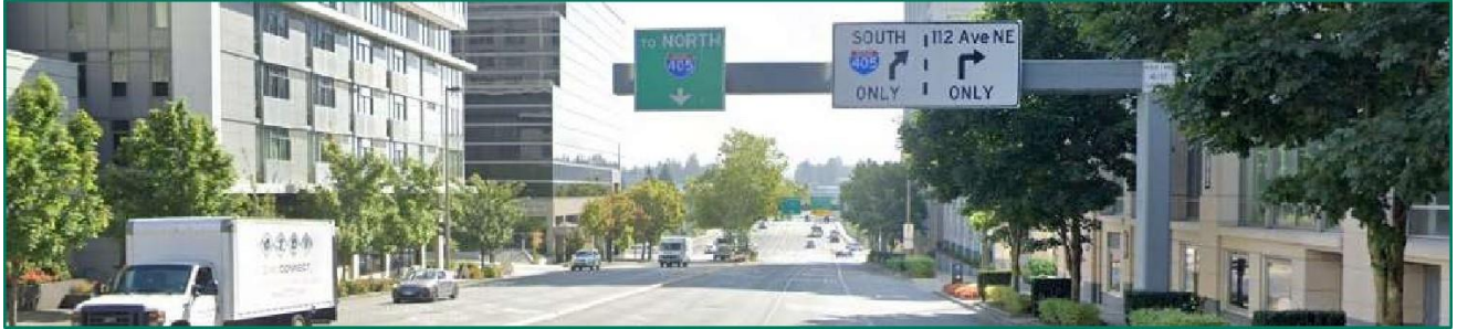
Cantilever arm: Single beam or support that extends horizontally from a fixed point without additional support underneath, allowing it to hold weight or carry loads (such as signs) at its free end. Pictured above: Cantilever arm on NE 8 th Street in Bellevue.
