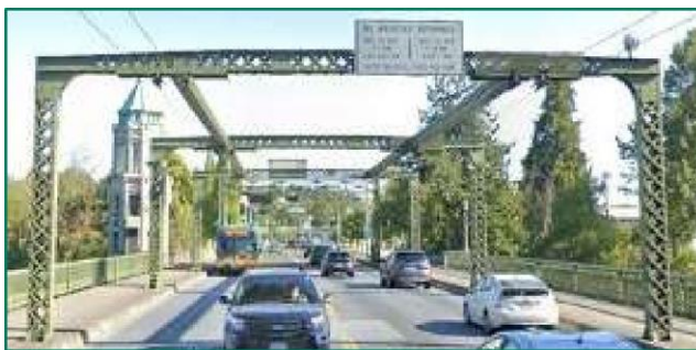
Use of existing structures (e.g., bridges and poles): Existing infrastructure used to hang signage. In the lefthand example above, the lattice-looking structure is part of the overall bridge design and serves multiple purposes in addition to supporting signage. Pictured above (left to right): Sign mounted on the Montlake Cut Bridge structure which also serves as trolley wire support; sign on a light pole on Brooklyn Ave NE in Seattle.
