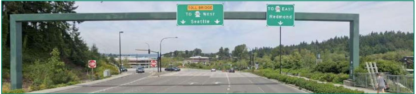
Sign bridge: Structure supporting signs spanning across a roadway. Pictured above: Sign bridge over Lake Washington Boulevard in Bellevue.
