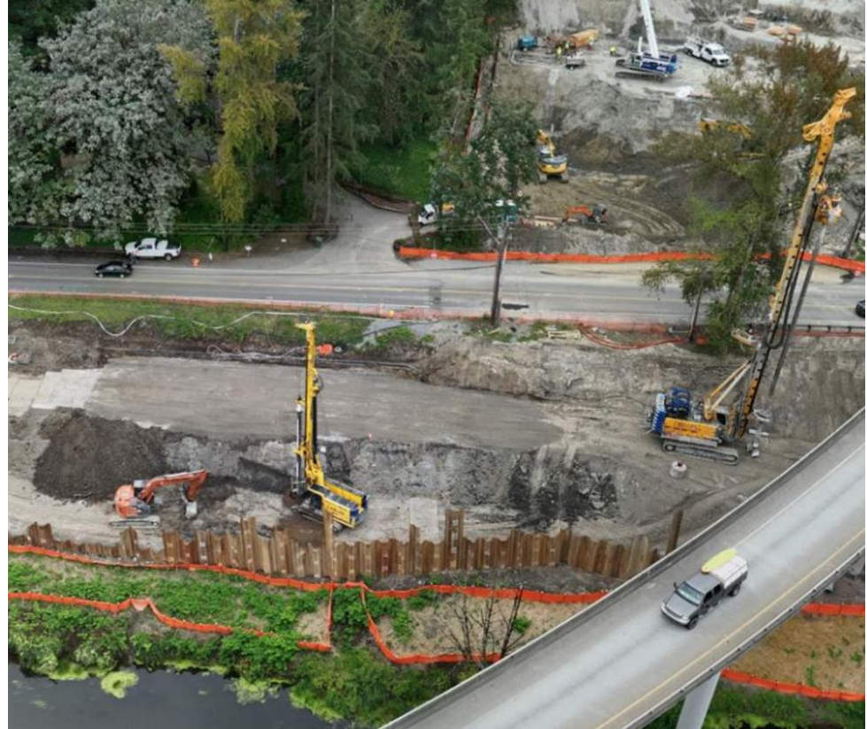
Looking south, crews work between the Sammamish River and Woodinville Drive
