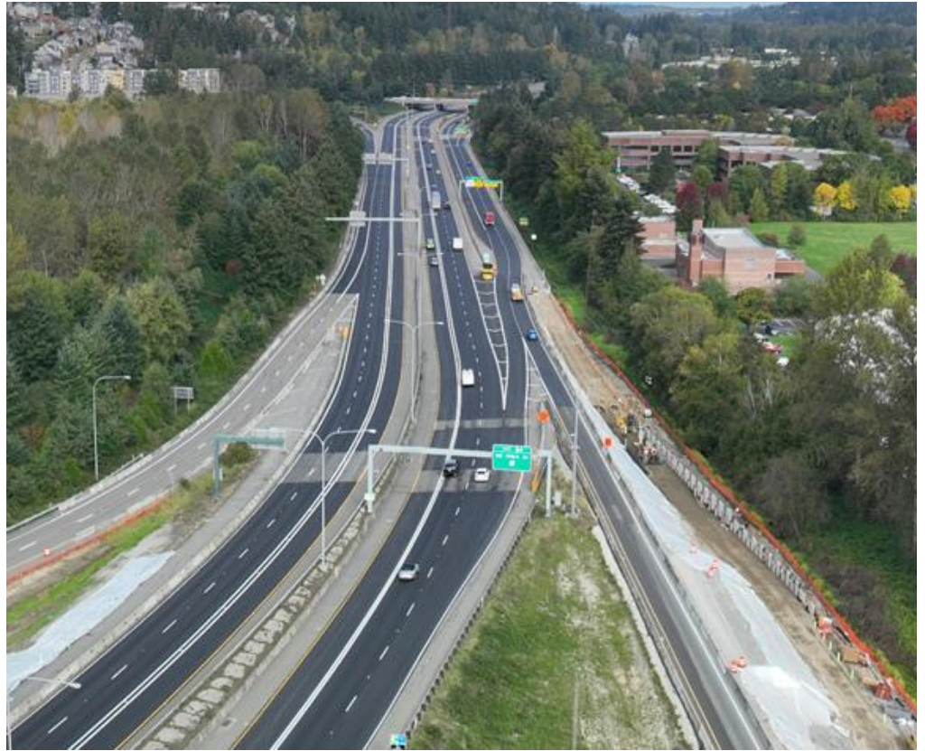
Looking north on I-405 at NE 195th Street
