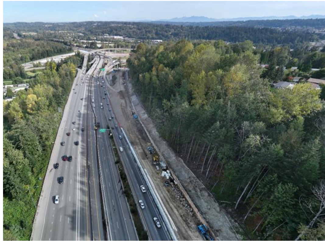
Looking north, soldier pile and tieback wall construction along northbound I-405
