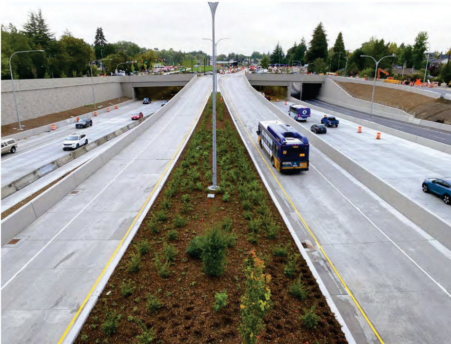
HOV direct access ramps (September 17)
