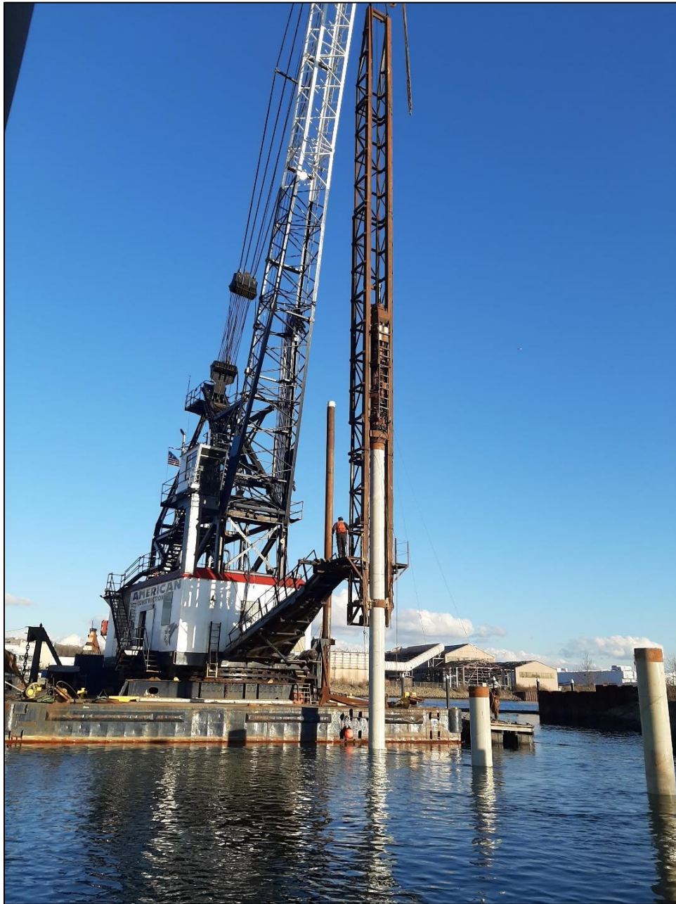
Photograph 1. Impact hammer configuration.
