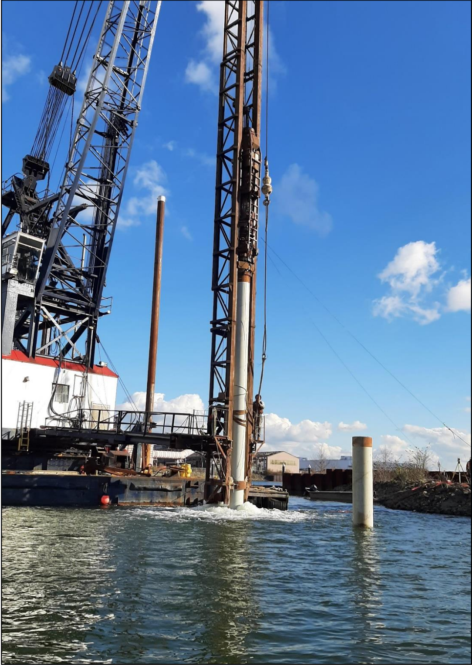
Photograph 3. Bubble curtain running during impact driving of pile P-05.
