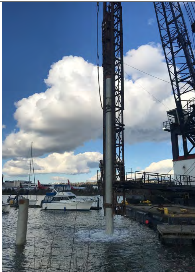
Plate 4 – Impacting pile P-05 on 2/9/21 using bubble curtain method. Looking northeast.
