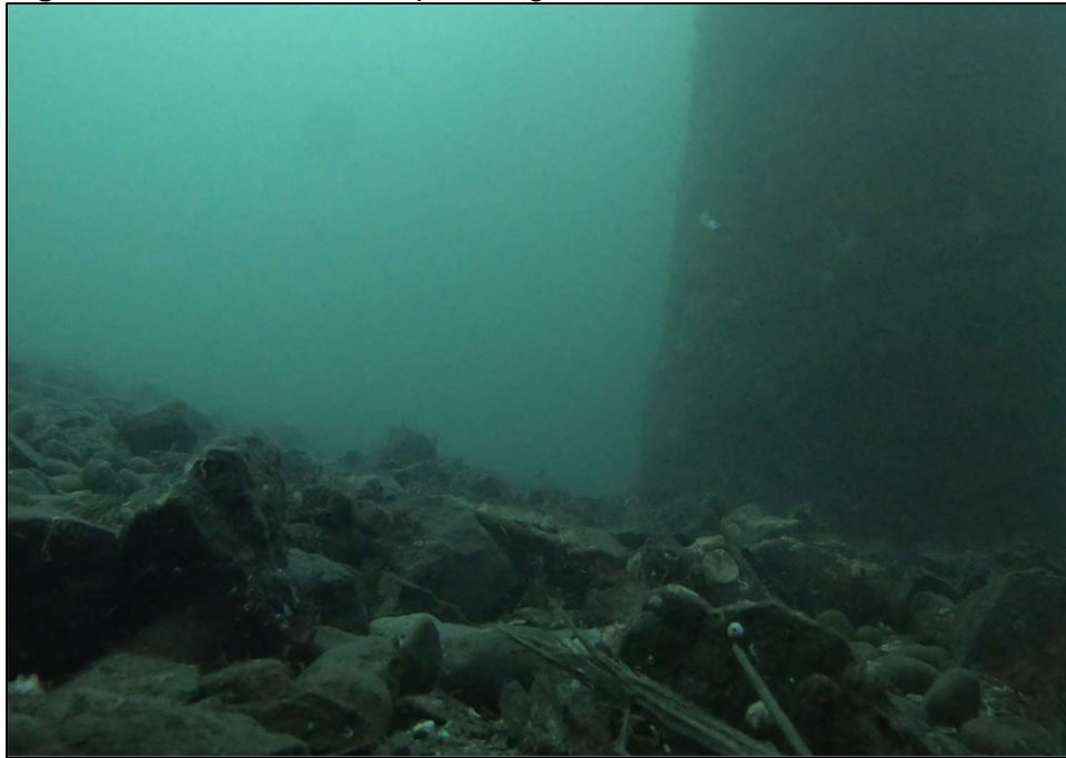
Figure 5.1 Seafloor Near Slip 2 Bridge Seat
