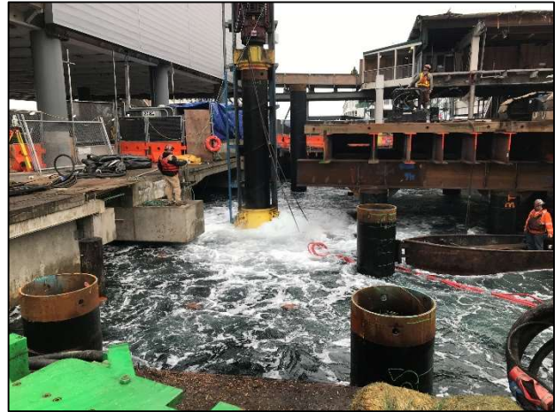
Figure 5.3 Operating Bubble Curtain
