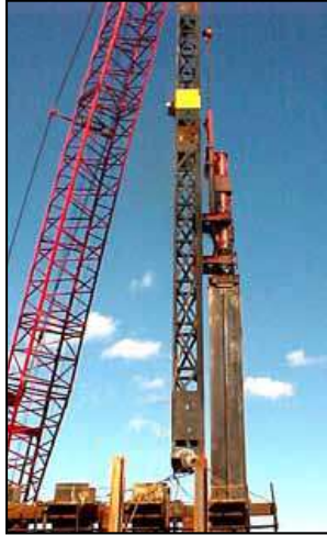
D62-52 in a stand-off driving Kingpile.
