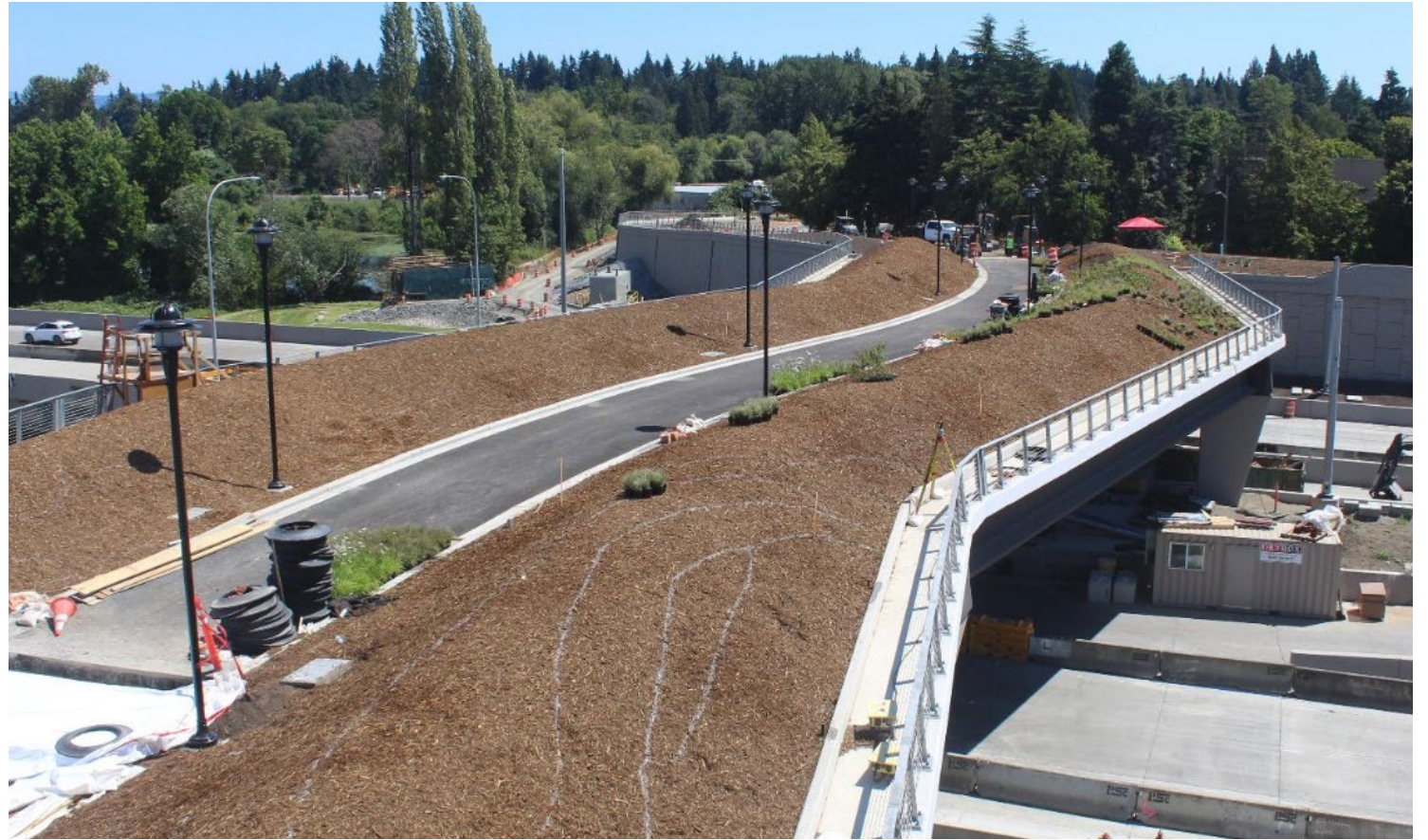
Bicycle and pedestrian bridge deck (June 26)
