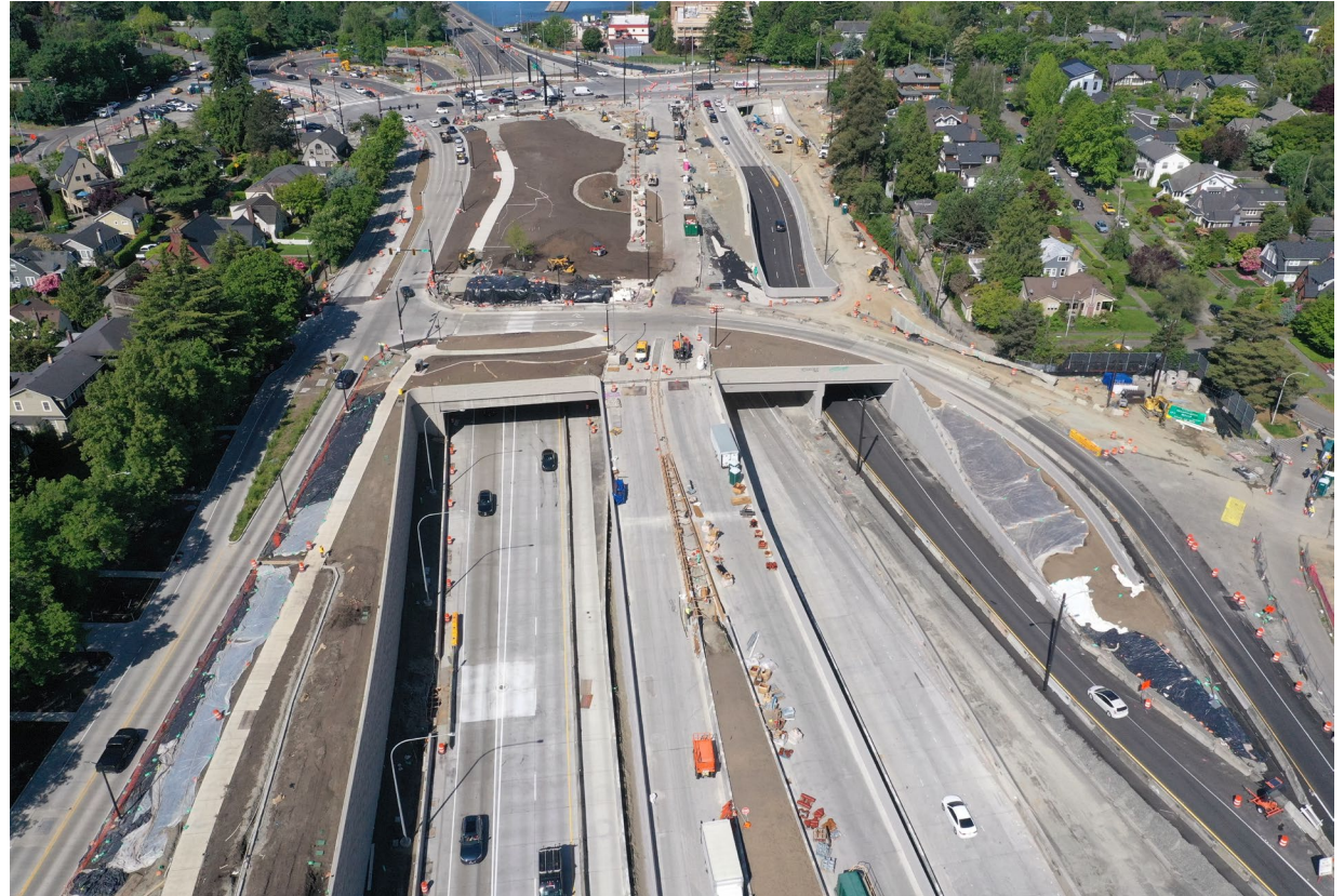
HOV direct access ramps (May 23)
