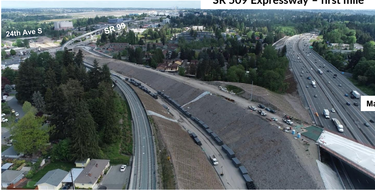
SR 509 Expressway – first mile
