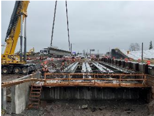
Bridge girder setting on SR 99.
