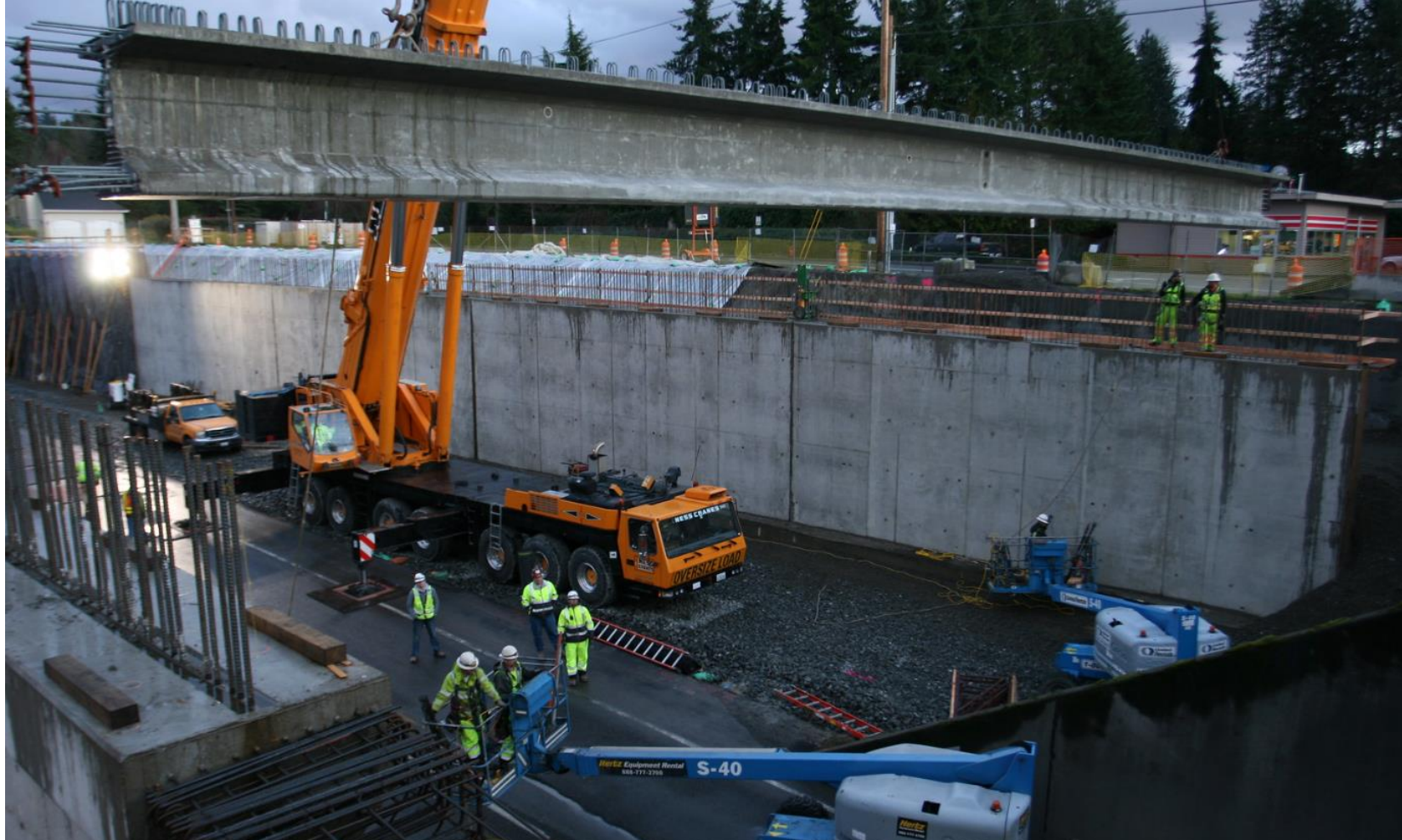
Example photo of girder setting
