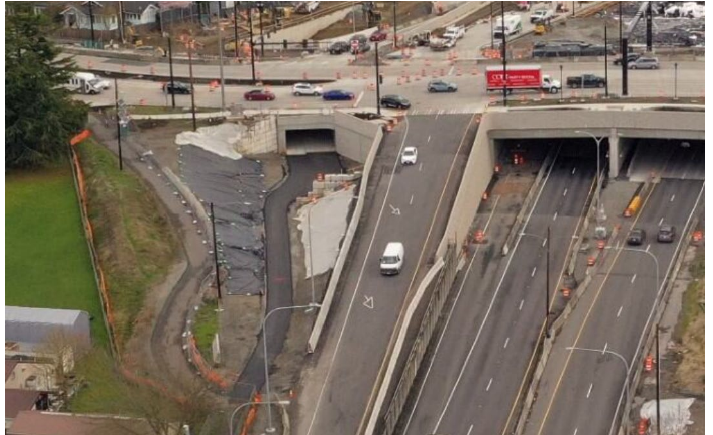
West entrance to the tunnel under Montlake Boulevard (March 26)
