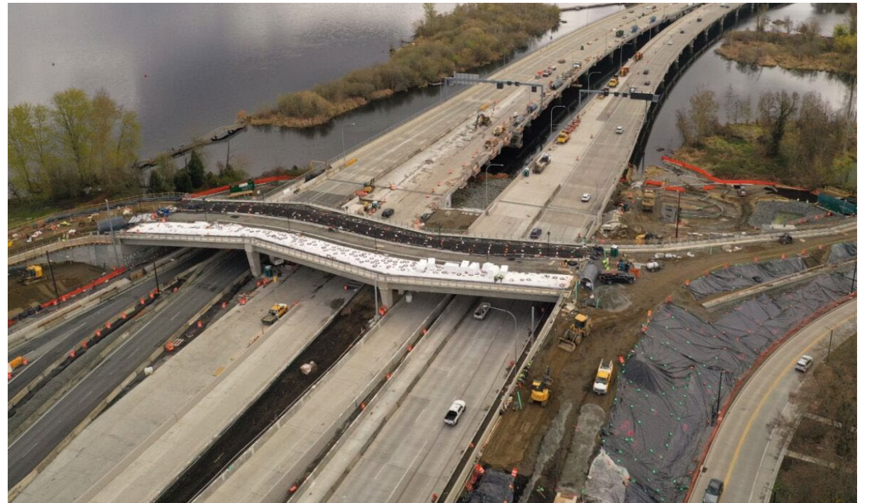
Bicycle and pedestrian bridge deck (March 26)
