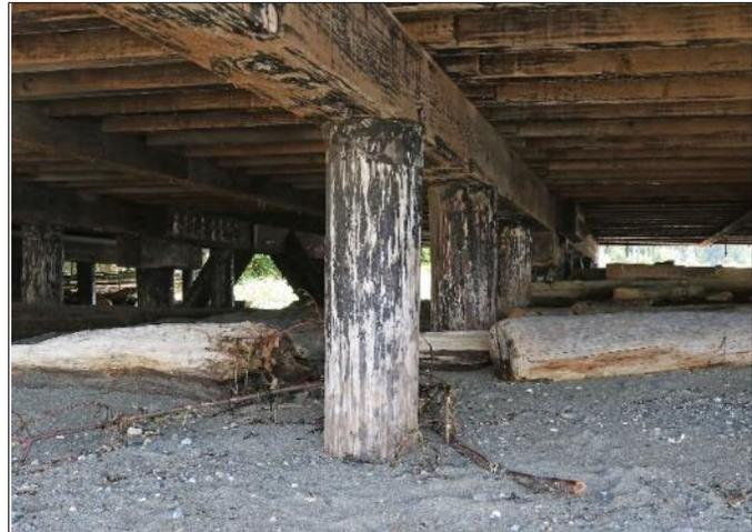
**Figure 1. Timber piles supporting the Terminal trestle**
