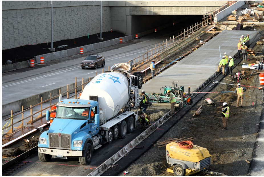
HOV direct access ramp paving. (Nov. 3)
