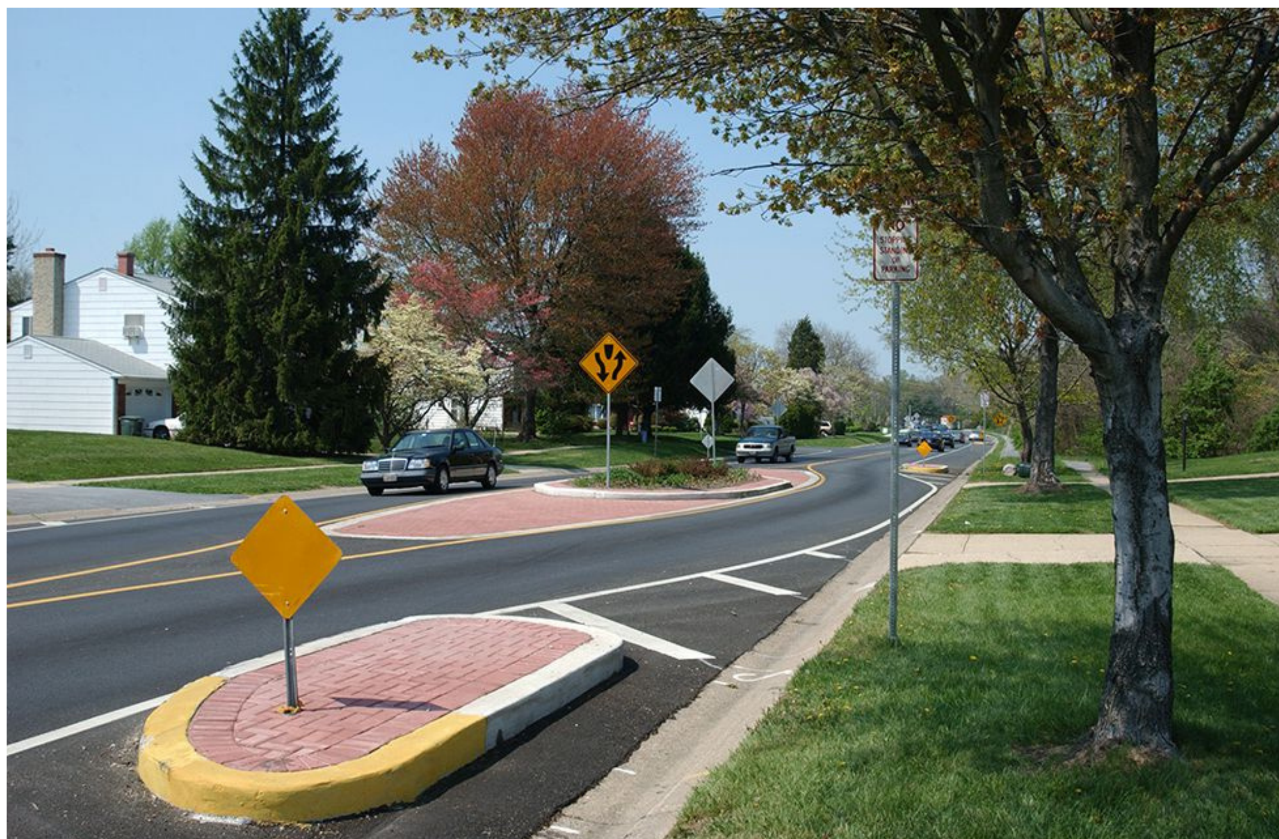
Example of a chicane using medians to shift the path of vehicles, slowing them down.
