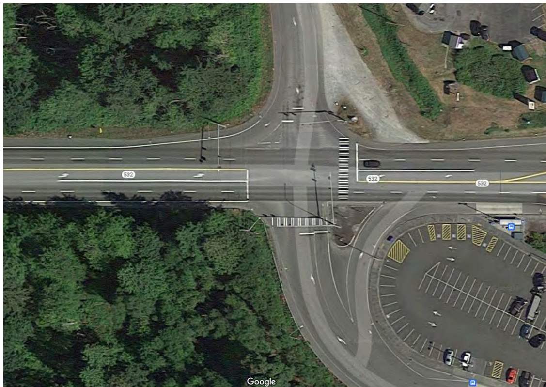
Figure 44. SR 532 and Old 99 North I/S at MP 9.94
