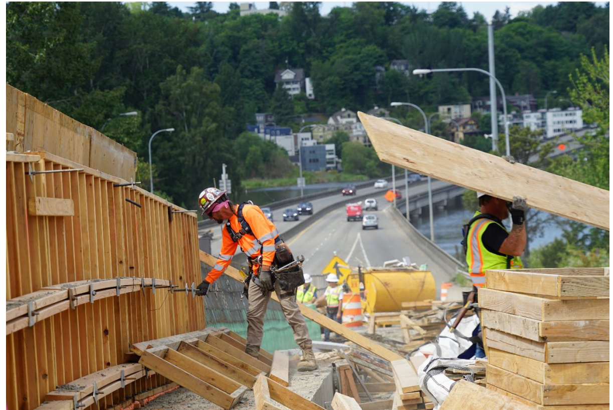
Barrier on the west end of the Montlake lid. (June 1)
