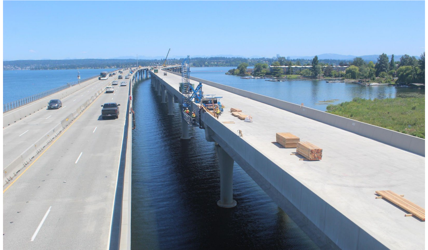
On the right is the new eastbound SR 520 bridge. (June 6)
