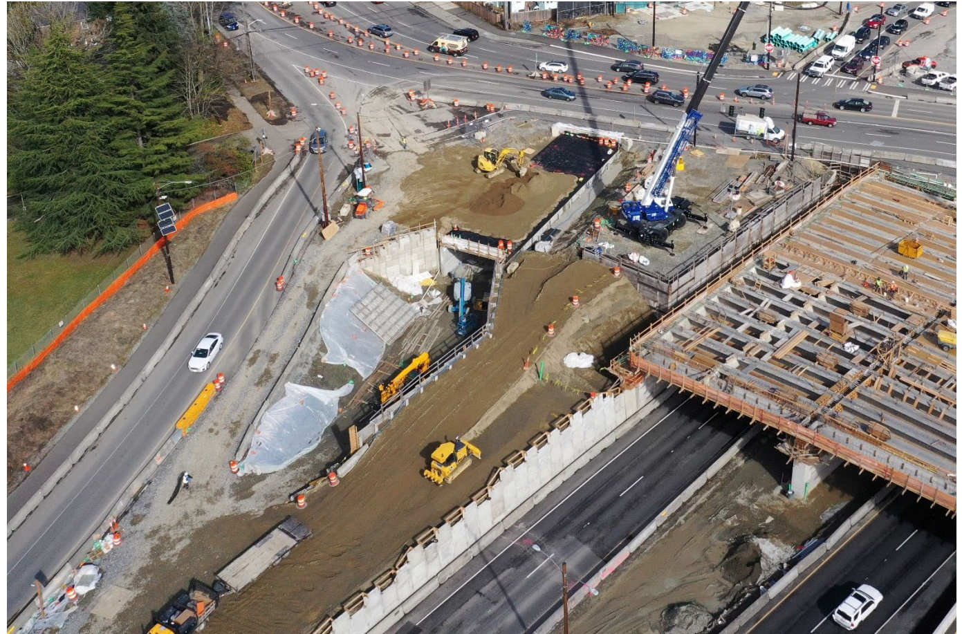
Girders installed for the HOV direct access ramps. (March 1)
