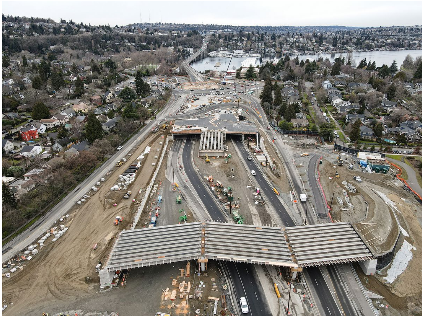
Looking west over the project area. (Feb. 26)
