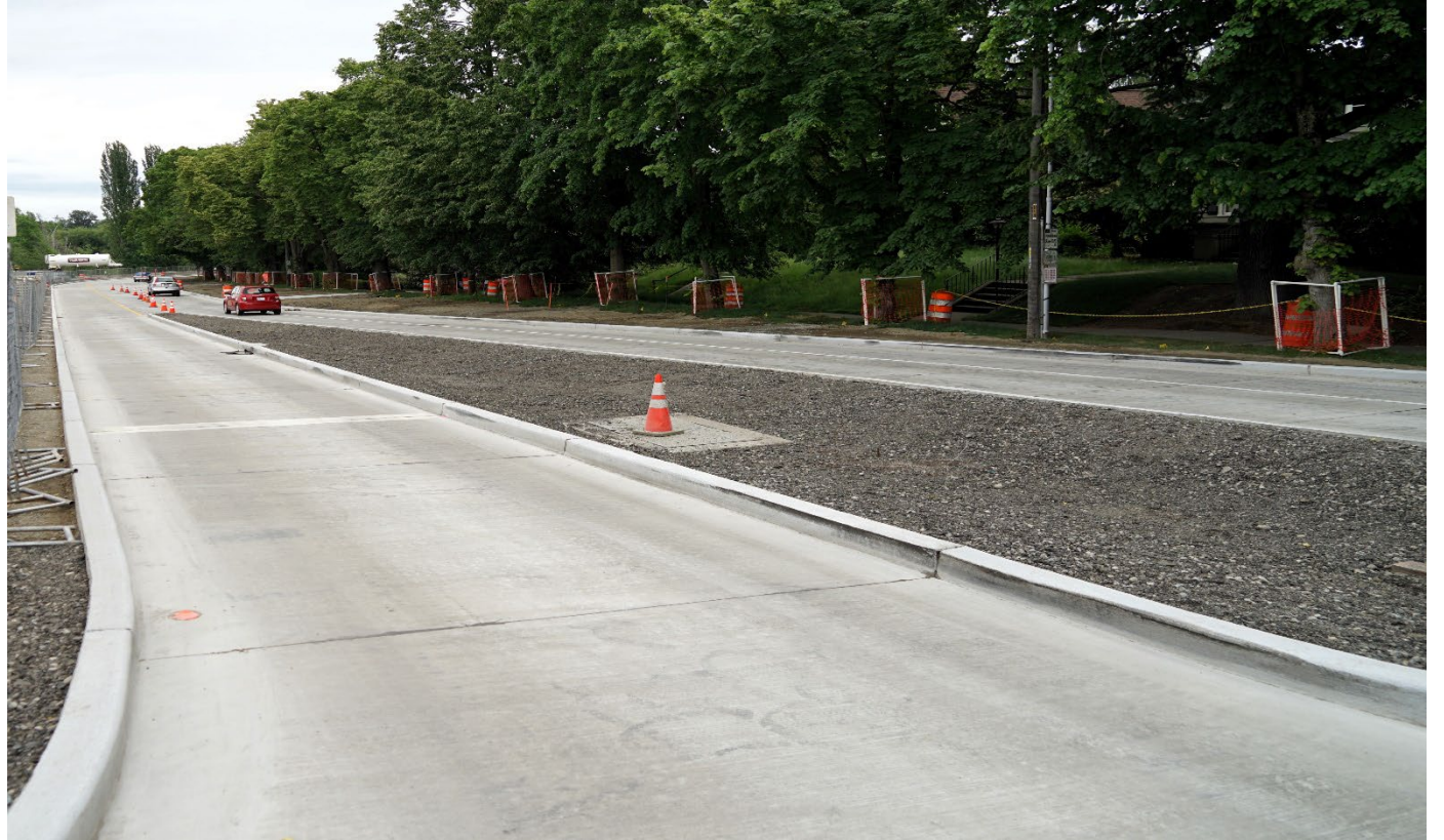
New Lake Washington Boulevard paving. (May 22)
