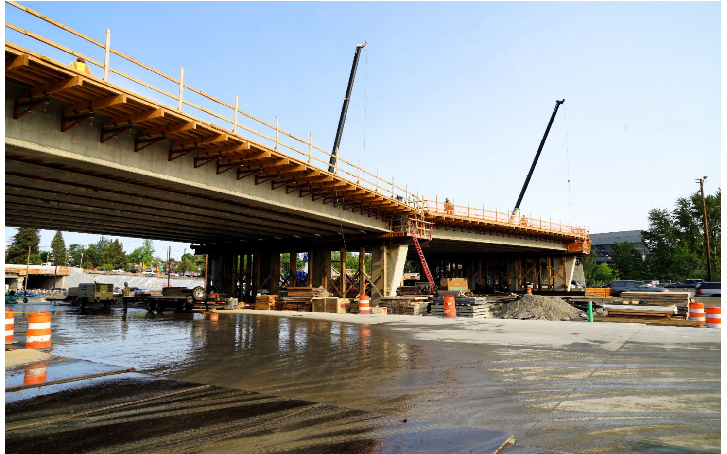
Bicycle and pedestrian bridge across SR 520. (May 17)
