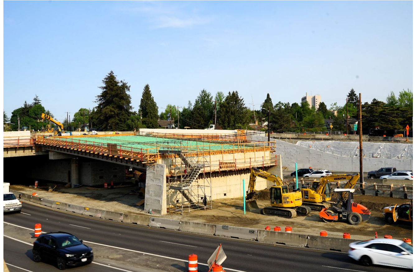
HOV direct access ramp. (May 17)
