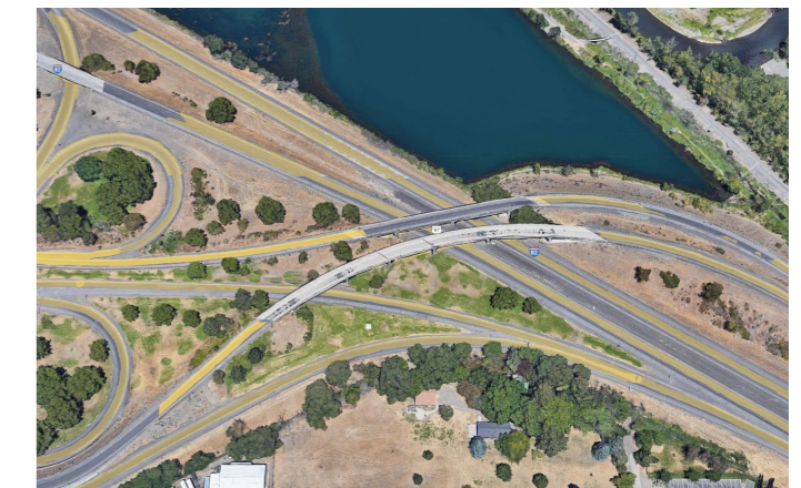
Bridge 82/118 W-S, north is to top of photo
