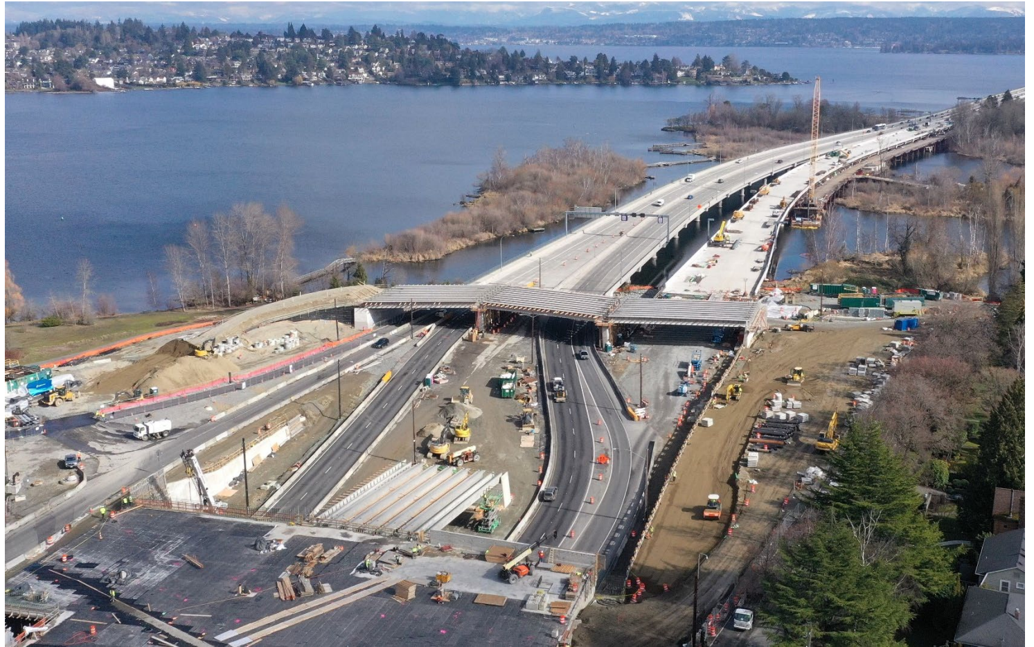
Girders installed for the bike and pedestrian bridge. (March 1)
