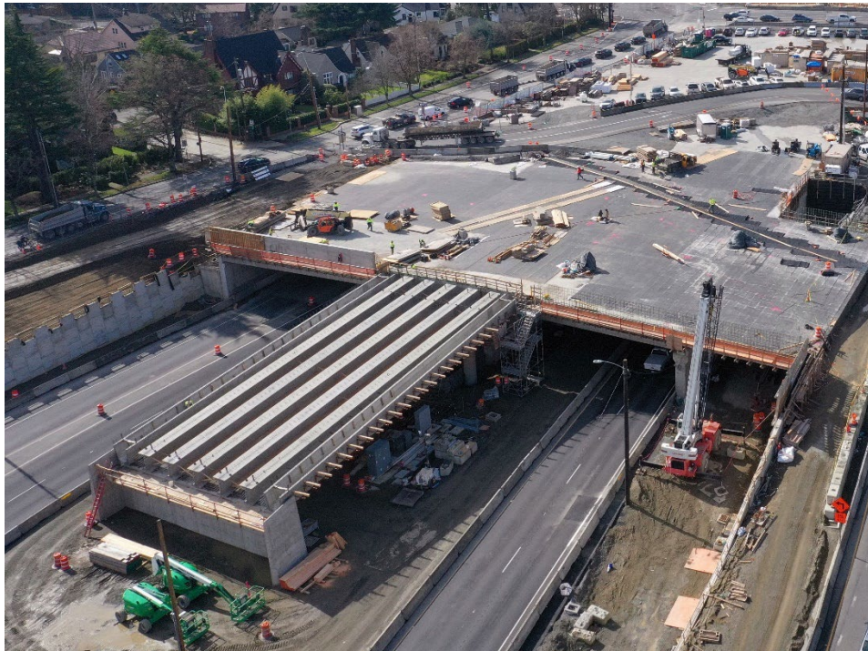
Girders installed for the HOV direct access ramps, (March 1)
