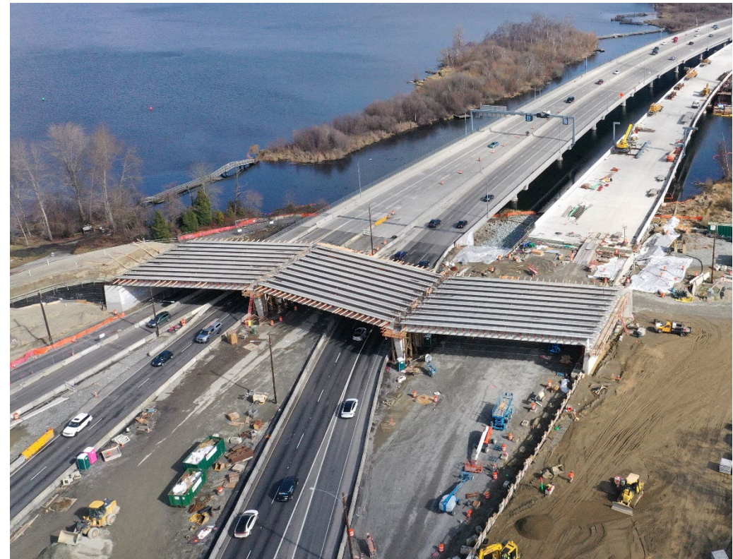
Girders installed for the future bicycle and pedestrian bridge (March 1)
