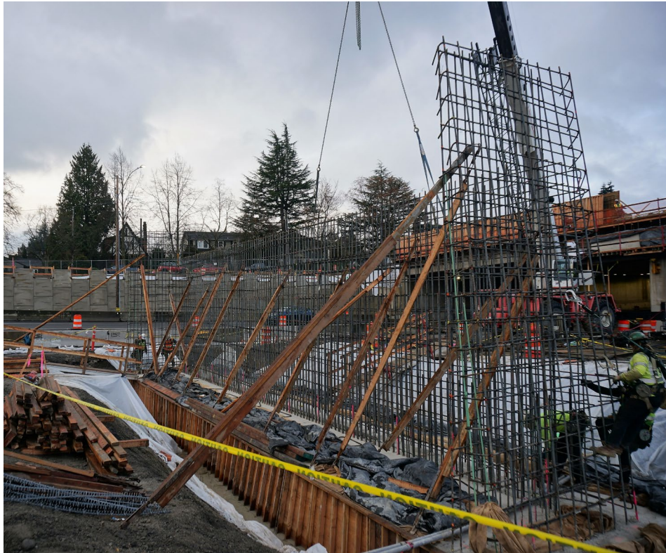
Crew constructing abutment for HOV direct access ramp. (Jan. 25)
