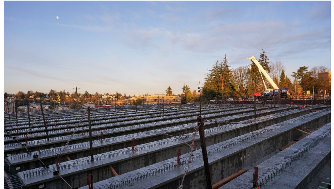
Girder placement on Montlake lid. (Jan. 10)
