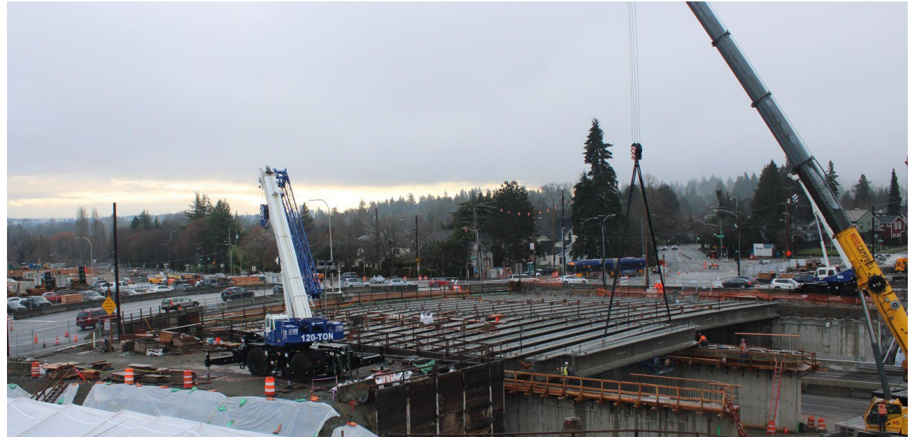
Final girders installation during the weekend of Jan. 20-23. (Jan. 22)
