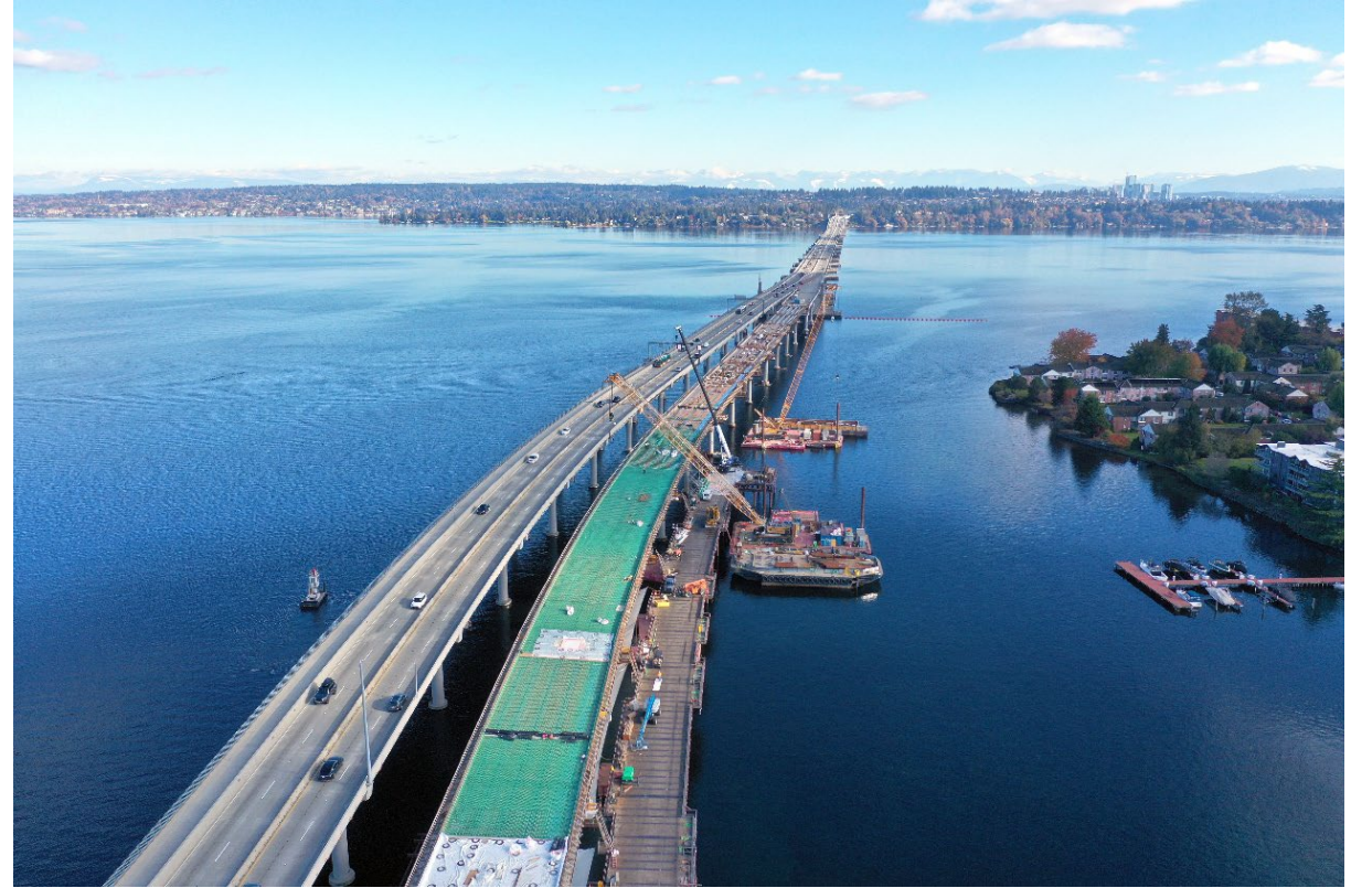
The green re-bar is installed prior to pouring concrete. (Nov. 9)
