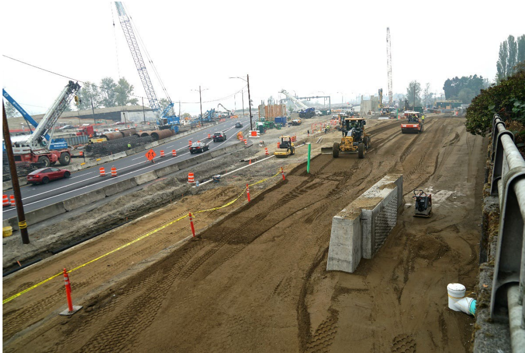
Soil compaction work north of Lake Washington Boulevard. (Oct.20)
