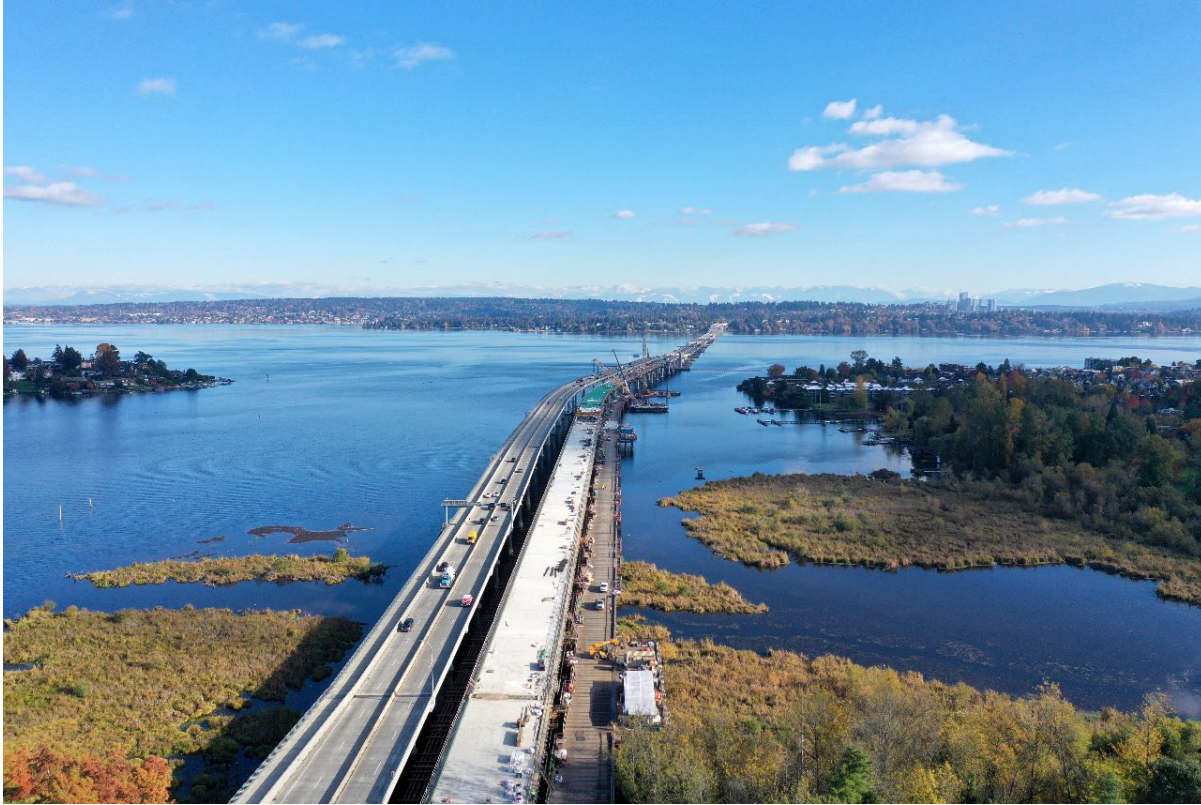
Completed concrete deck paving is the white area. (Nov. 9)
