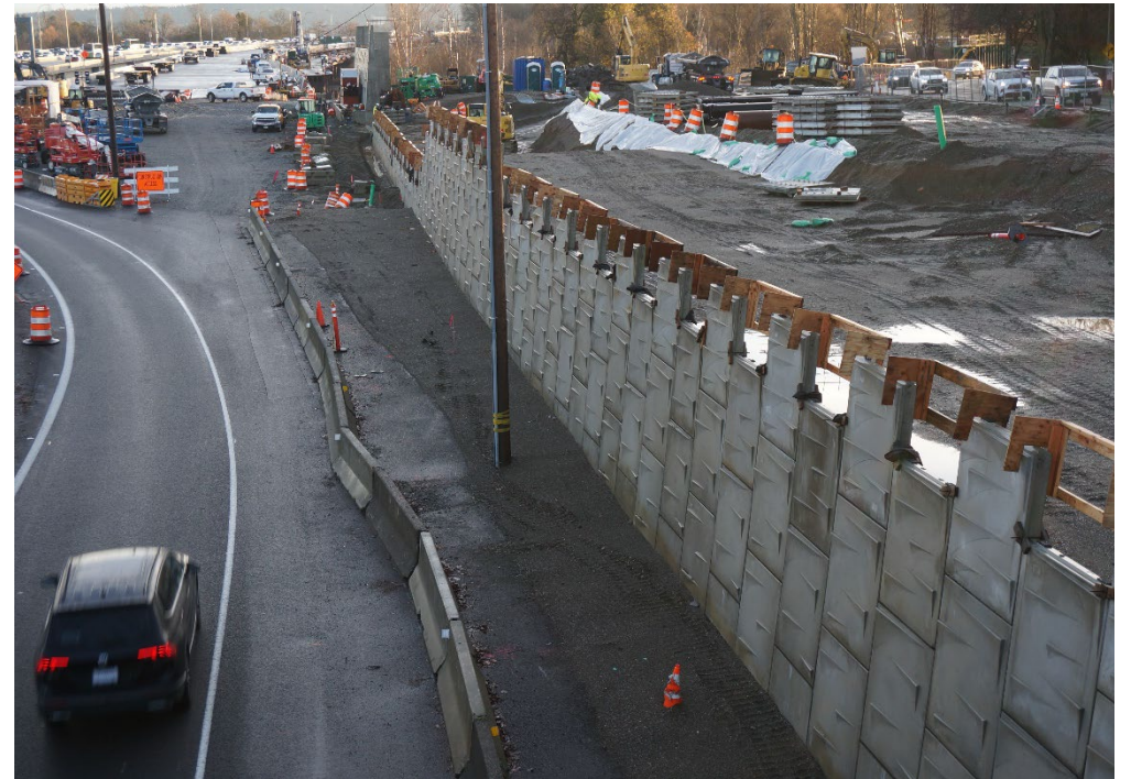
View of retaining wall construction north of Lake Washington Boulevard. (Jan.10)
