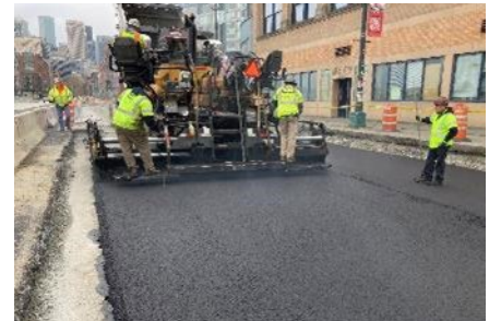
HMA paving on 1st Ave S.
