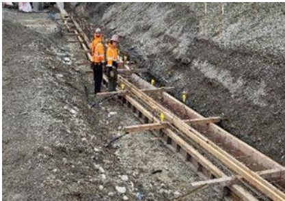
Wall SW- 36 formwork rebuilding
