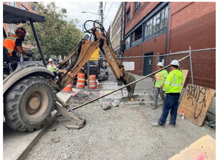
9/14/22: Signal pole excavation at the corner of South Dearborn Street and First Avenue South.
