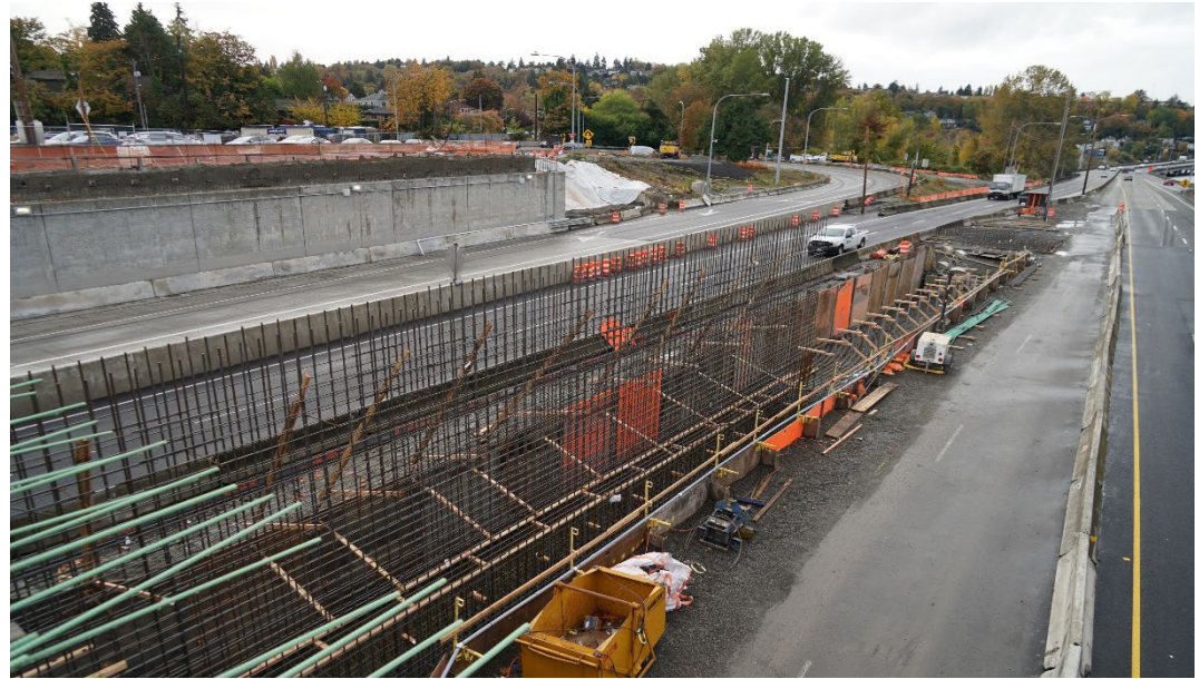
Preparing for 2023 girder installation on the west side of the Montlake lid. Pier 2 is under construction in the center of the roadway. (Nov. 1)
