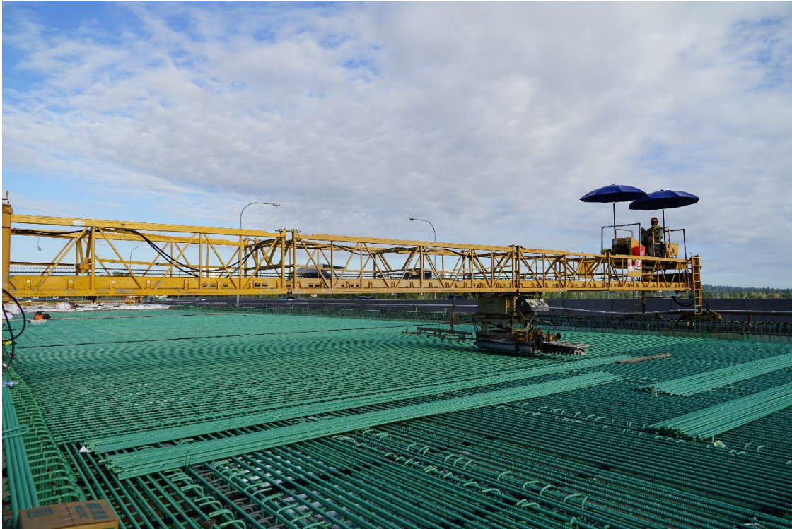
Green rebar will reinforce the concrete bridge deck.
