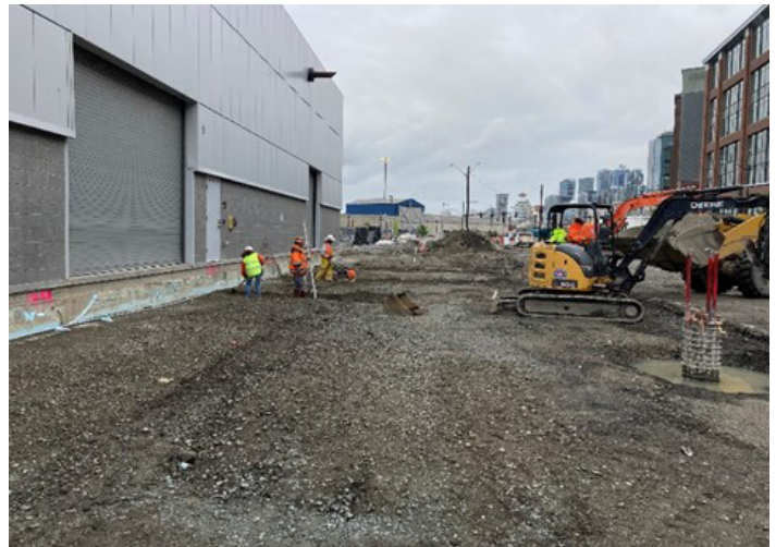
5/6/22: Excavation for grade beams for the equipment garage
