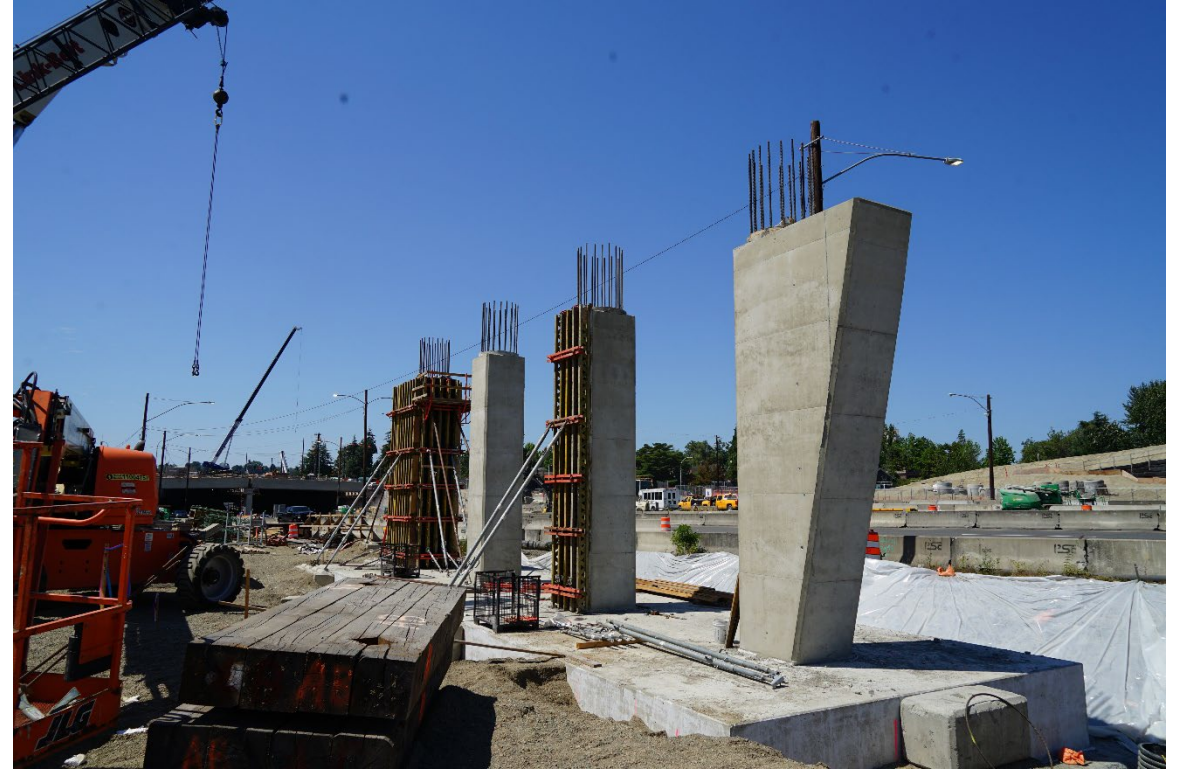
Crews are constructing part of the bridge on the south side of SR 520 along Lake Washington Boulevard.
