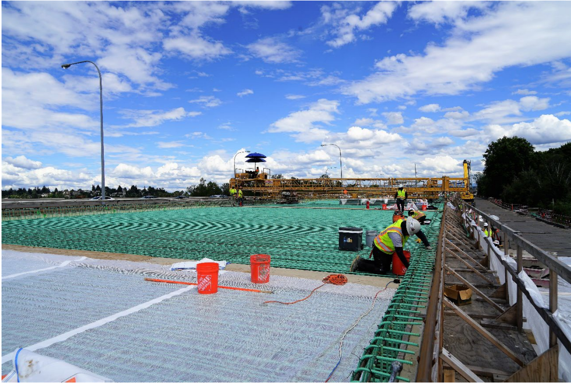
Crews wire together rebar to reinforce the bridge deck prior to pouring concrete.
