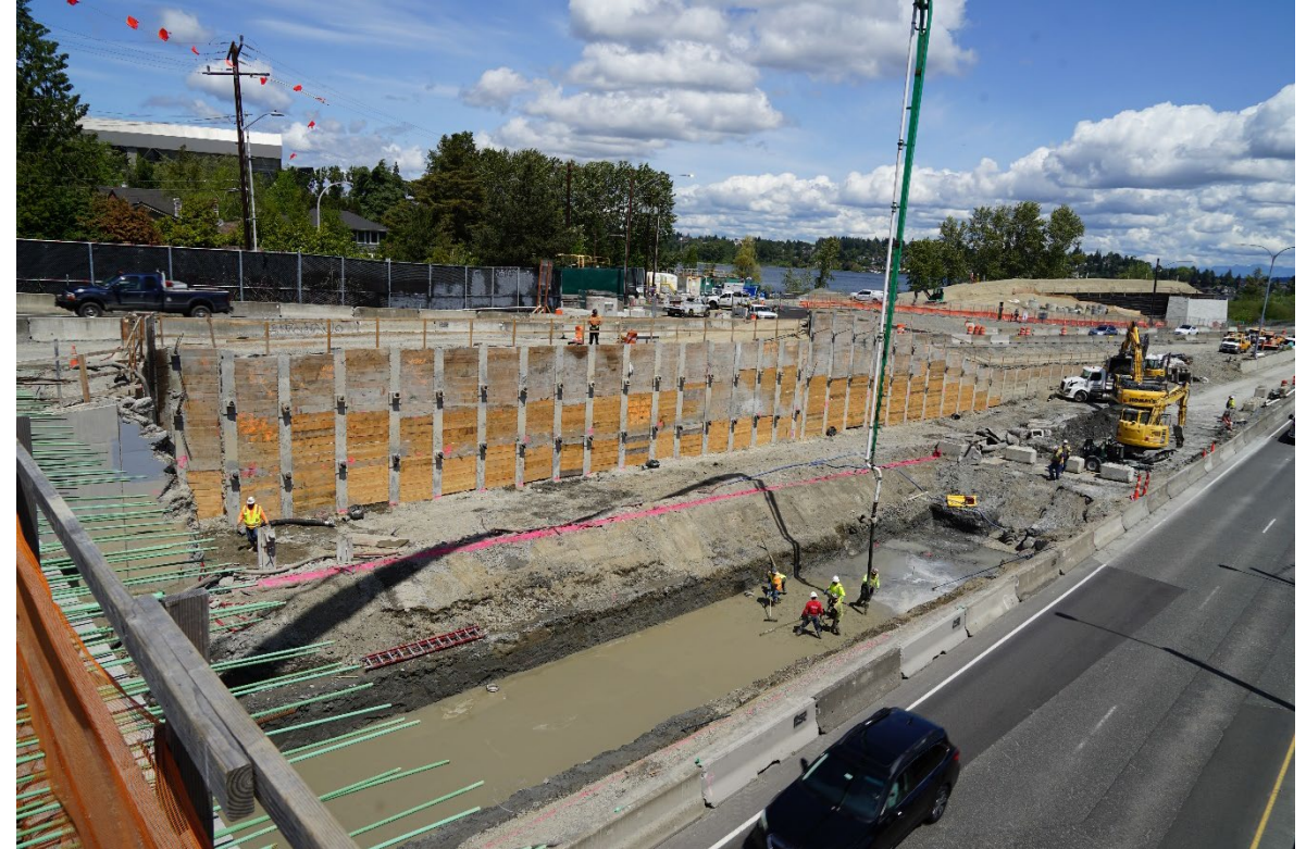
Pier 3 east with pier 4 foundation being poured in foreground
