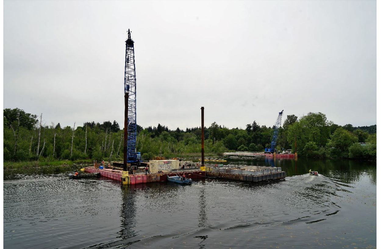
Crew on crane barge completing removal of the old on-ramp
