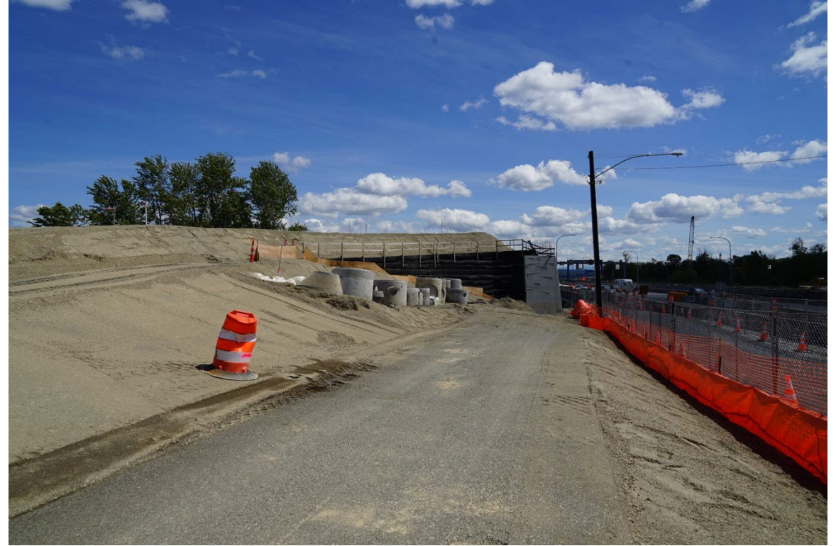
Crews are constructing an embankment for the bridge in East Montlake Park.
