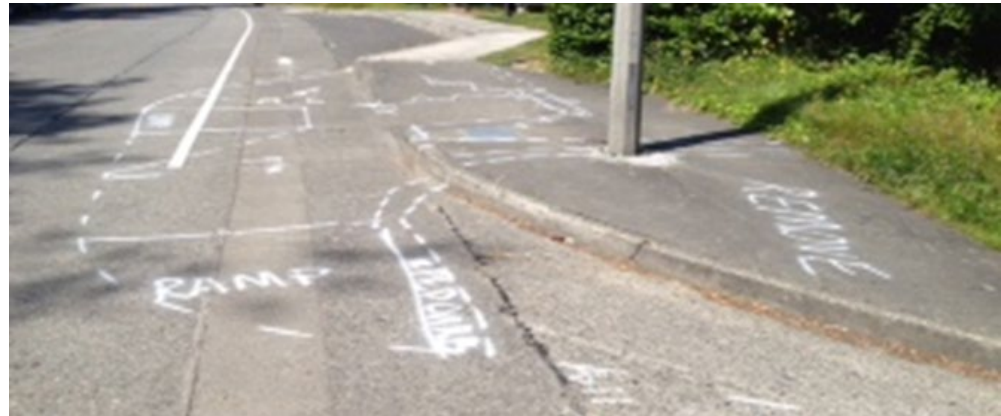
A curb and sidewalk that have been marked with white paint to indicate where a new curb extension and curb ramp will be installed.
