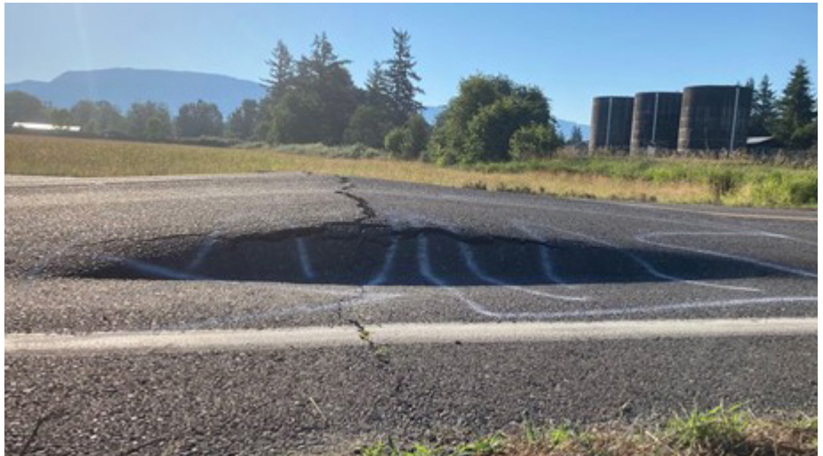
Extreme heat during the 2021 summer resulted in pavement buckling on SR 544 in Whatcom County.
