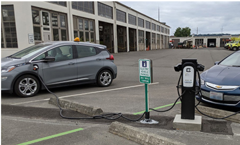
WSDOT's Northwest Region Corson Avenue building level 2 chargers are in operation. WSDOT installed six level 2 chargers and two DC fast chargers at this site.
