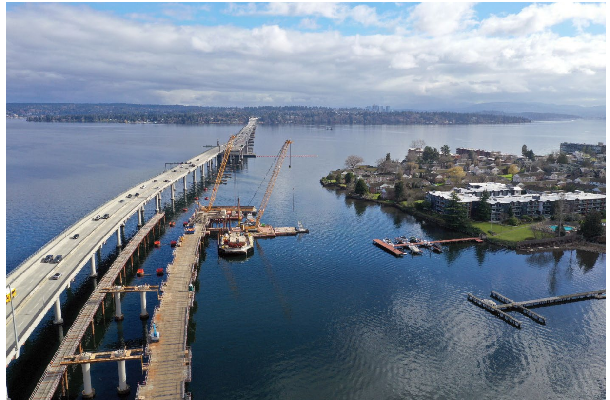
Construction of new eastbound bridge.
