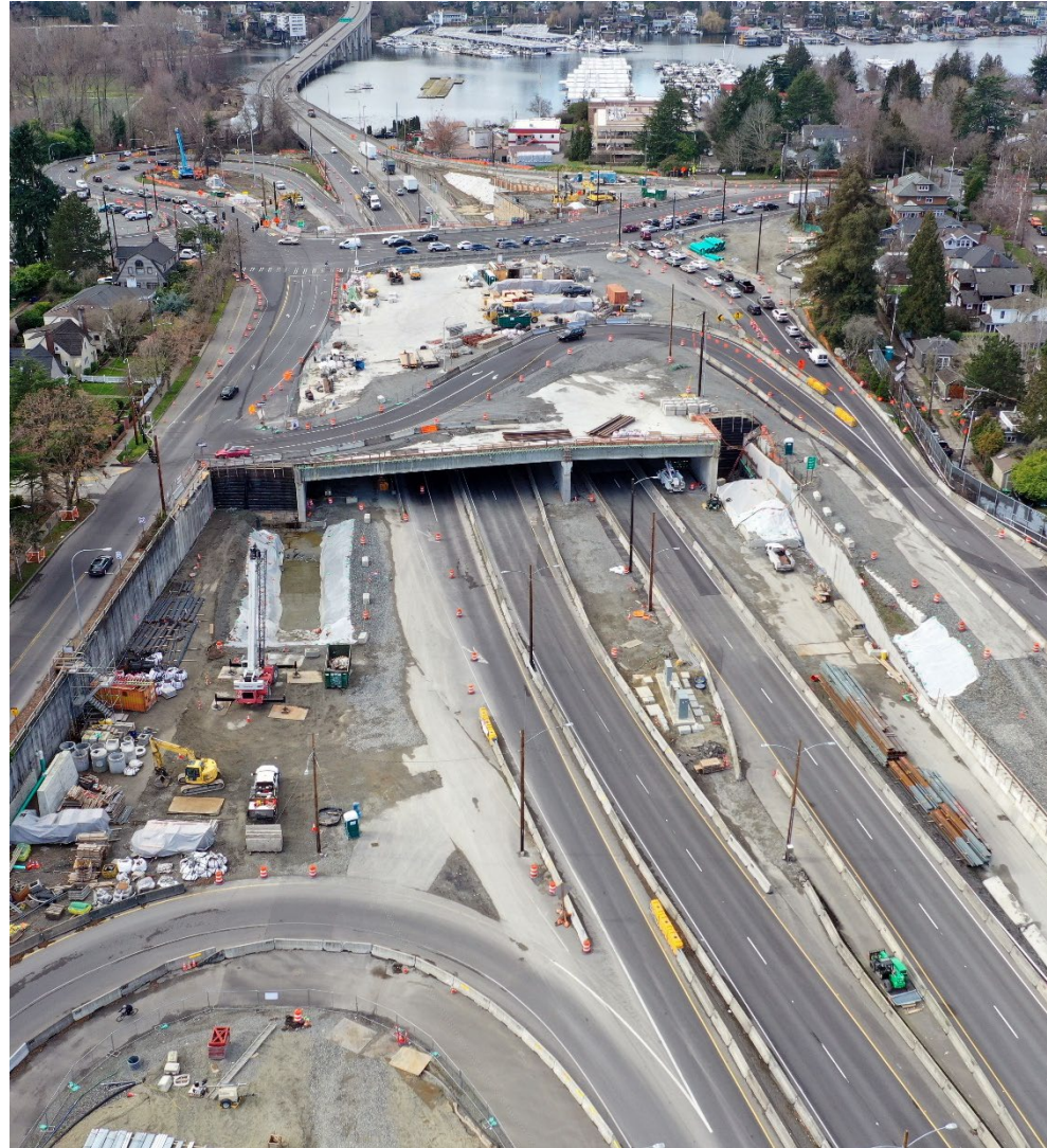
Construction of the Montlake lid. Looking west toward Portage Bay.
