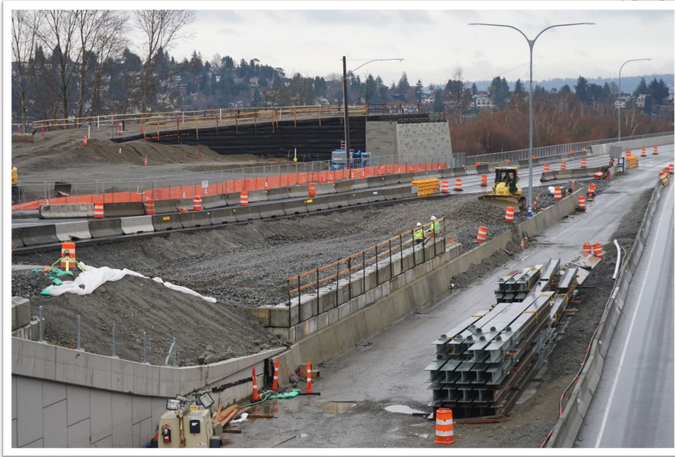
Location of future supporting wall, looking northeast from the lid.
